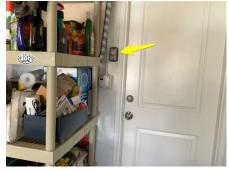
**CR 149:** An extension cord is being used to supply electricity to the garage door opener. We suggest a qualified garage door technician should install a proper receptacle to serve the garage door opener.
