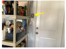
**CR s-149**: An extension cord is being used to supply electricity to the garage door opener. We suggest a qualified garage door technician should install a proper receptacle to serve the garage door opener.
