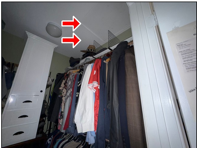
3.3 Item 1 (Picture) Structural Components
