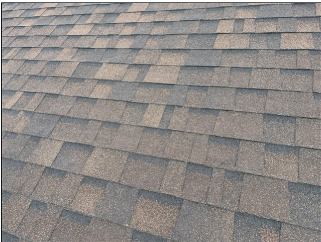
1.0 Item 2 (Picture) Roofing
