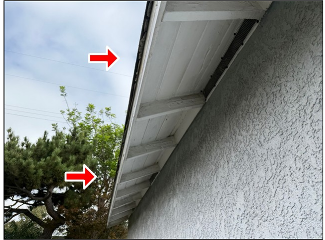
1.3 Item 2 (Picture) Roofing
