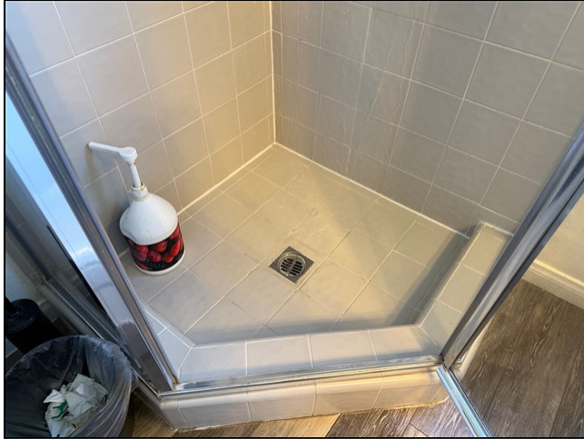
8.9 Item 1 (Picture) Interiors
