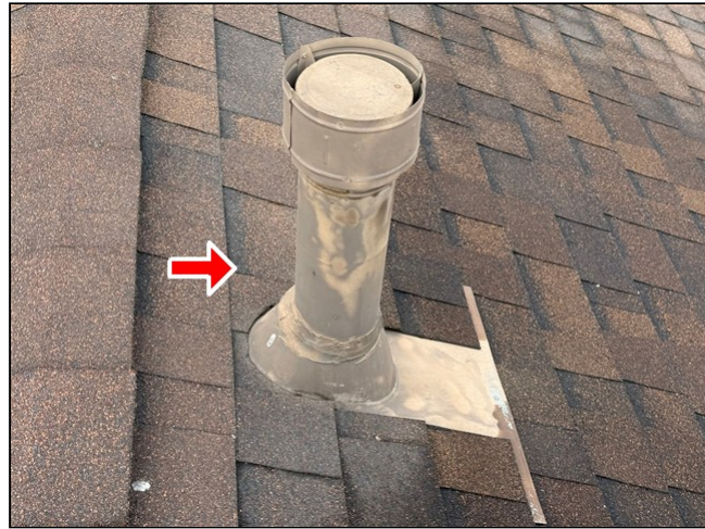
Item 1 - Item 2 (Picture) Roofing
