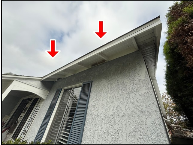
1.3 Item 1 (Picture) Roofing
