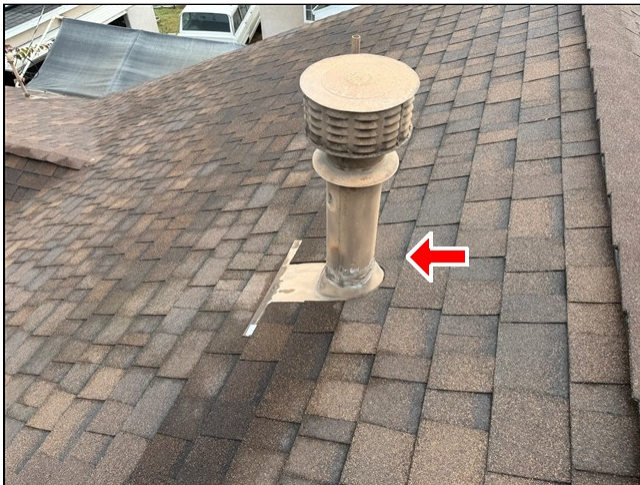
1.1 Item 1 (Picture) Roofing
