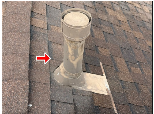
1.1 Item 2 (Picture) Roofing
