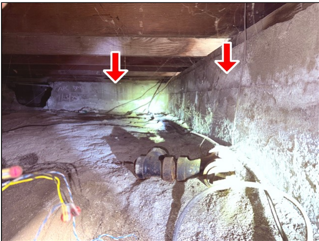
3.0 Item 2 (Picture) Structural Components
