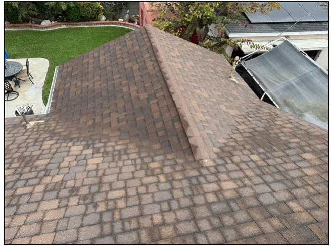
1.0 Item 4 (Picture) Roofing
