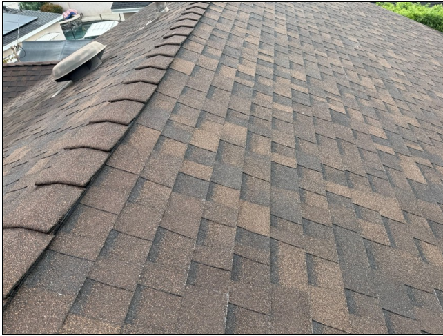
1.0 Item 3 (Picture) Roofing
