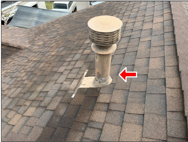
Item 1 - Item 1 (Picture) Roofing
