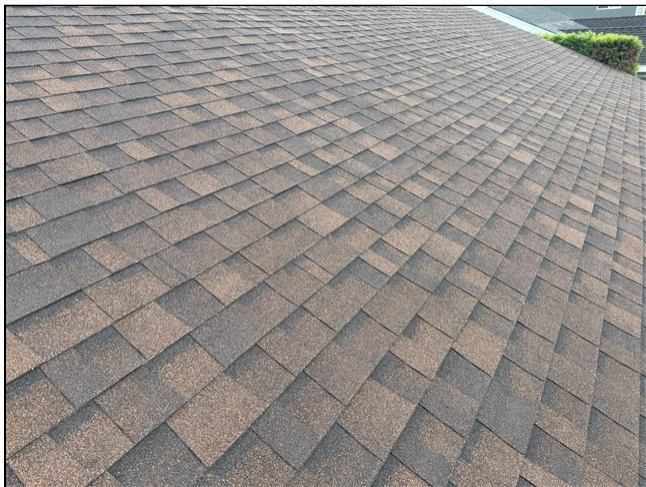
1.0 Item 1 (Picture) Roofing
