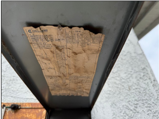
6.0 Item 3 (Picture) Electrical System
