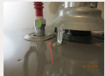
Distorted plastic bushing
