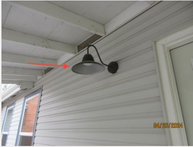
Rear of the house
