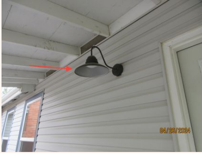
Rear of the house
