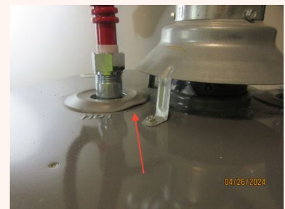
Distorted plastic bushing
