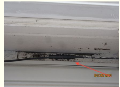
Left side of the house
