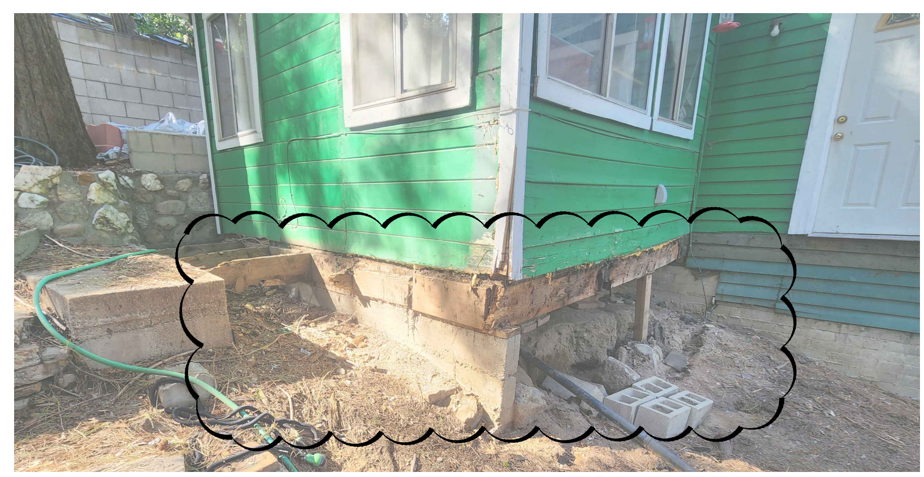
EXISTING EXPOSE FOOTING & STRUCTURAL VIEW
