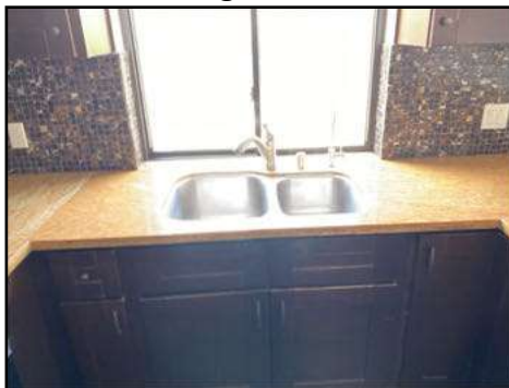
Gap at back splash to counter top joint - needs to be sealed to prevent unwanted moisture entering the cabinet
