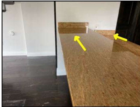
Gap at back splash to counter top joint - needs to be sealed to prevent unwanted moisture entering the cabinet
