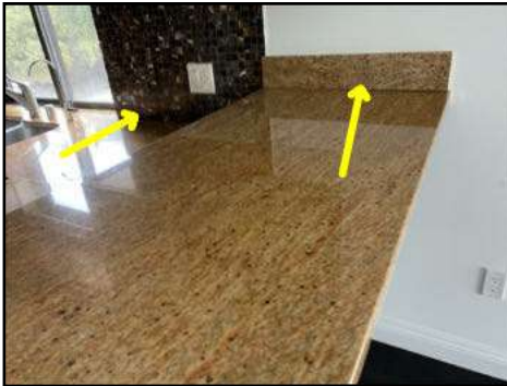
Gap at back splash to counter top joint - needs to be sealed to prevent unwanted moisture entering the cabinet
