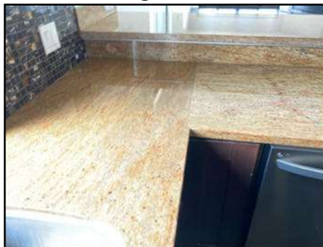
Gap at back splash to counter top joint - needs to be sealed to prevent unwanted moisture entering the cabinet
