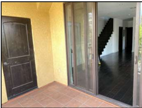
Door(s) swing outward with hinges exposed to the exterior (possible security concern) - recommend installing security hinges/pins to prevent easy removal
