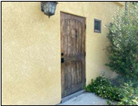
Door(s) swing outward with hinges exposed to the exterior (possible security concern) - recommend installing security hinges/pins to prevent easy removal
