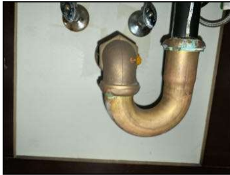
Older style metal traps present - traps can leak at any time due to corrosion
