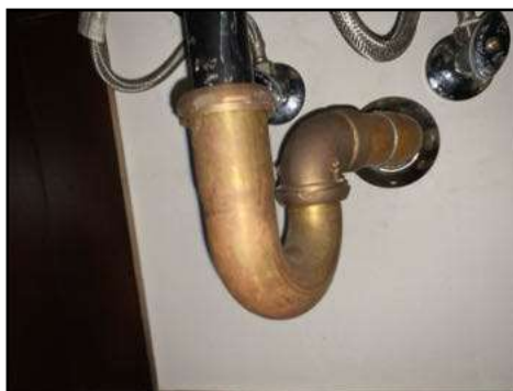
Older style metal traps present - traps can leak at any time due to corrosion
