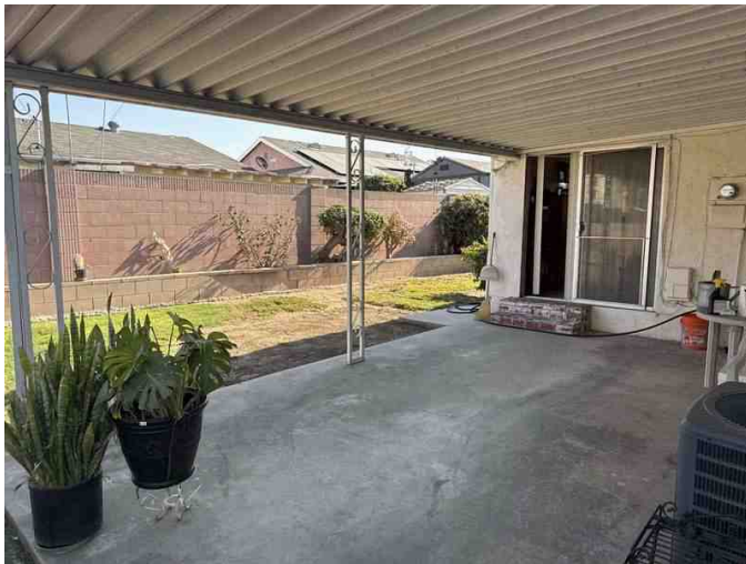
Rear Yard Pic
