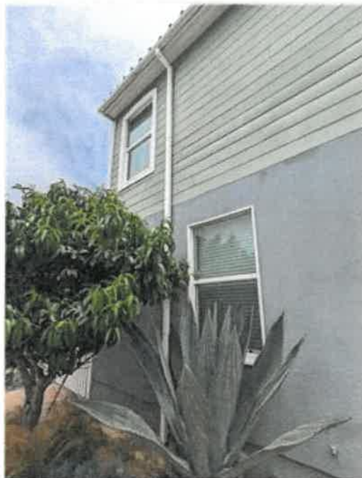
Downspout Front Of House
