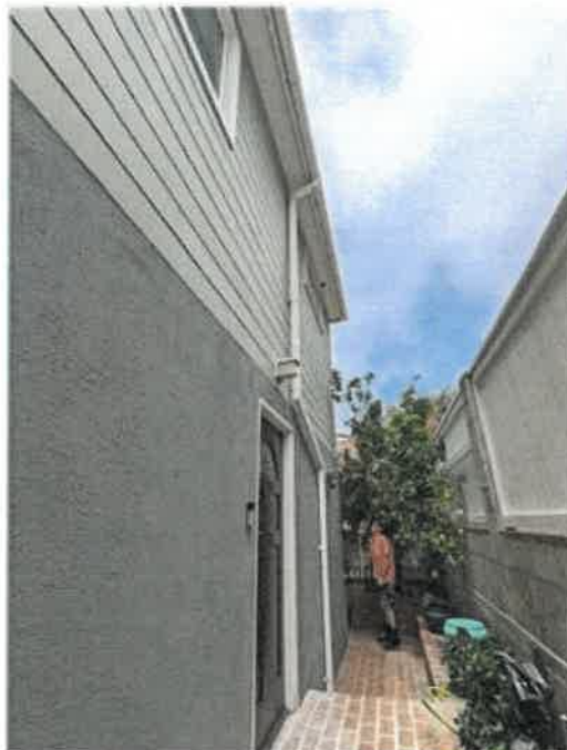
Downspout Back Of House
