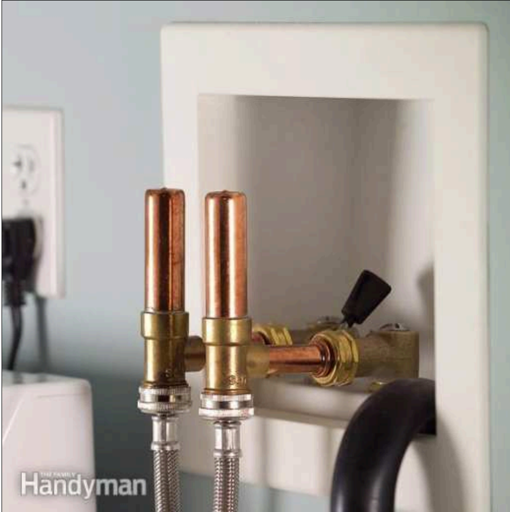
7.7 Item 1(Picture) HV
