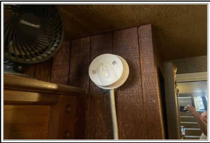
TYPICAL COMBO SMOKE / SMOKE DETECTOR
