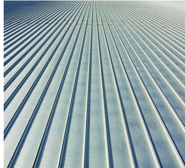
STANDING SEAM ROOF
