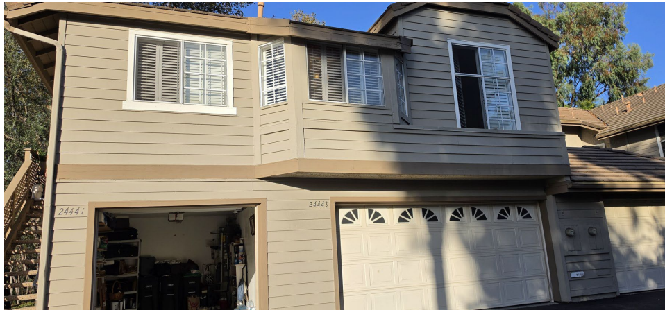
Exterior elevation showing the garage below the living-level floor; no cracking or distress observed at the exterior walls.
