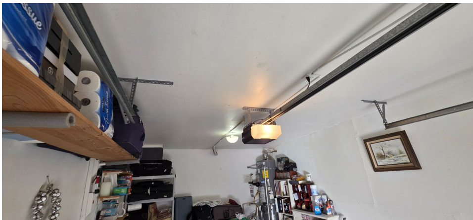
Garage ceiling and wall junctions toward the garage interior; no structural distress observed.
