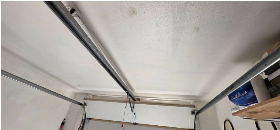
Garage ceiling below the living-level floor; the finish is continuous with no sagging, cracking, or separation observed.
