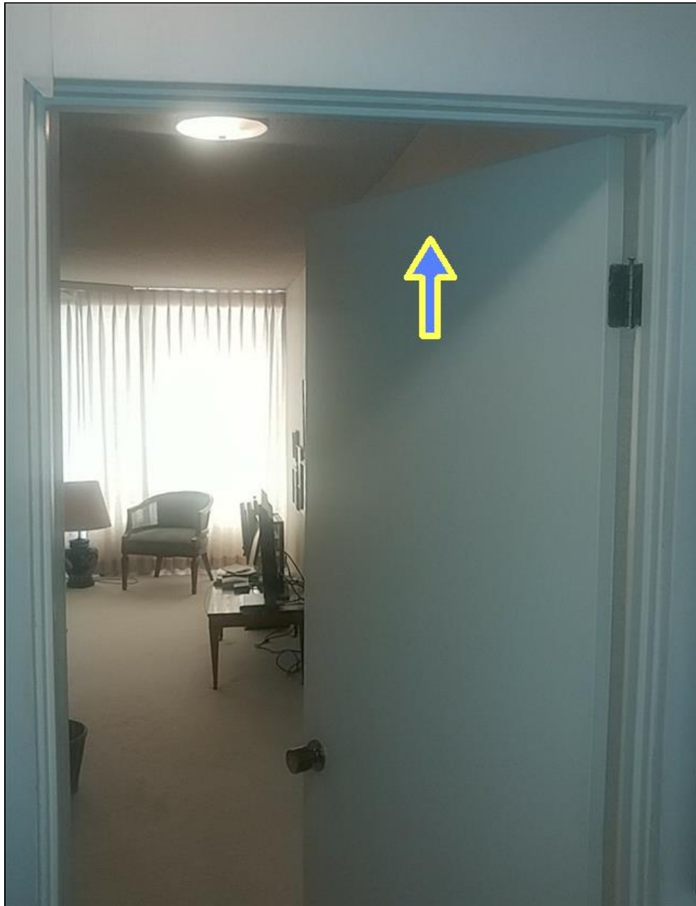
7.0.B Item 1(Picture) Bedroom door rubs and should be Serviced.
