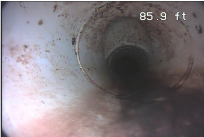
Drain waste pipe connection
