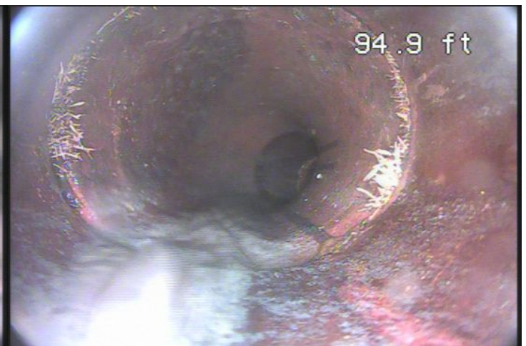
PVC to ABS pipe connection
