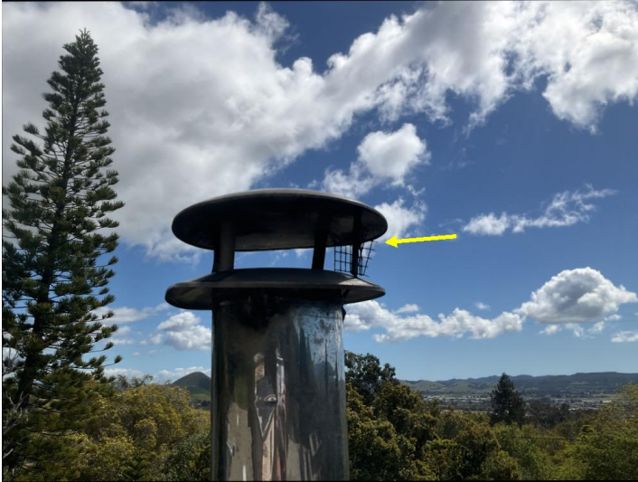
There is no spark arrestor on the chimney, which is required by current standards, and should be installed.
