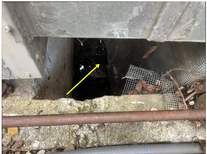
The ducts, as they enter the crawlspace, are in water. The duct will deteriorate more quickly and should be served.
