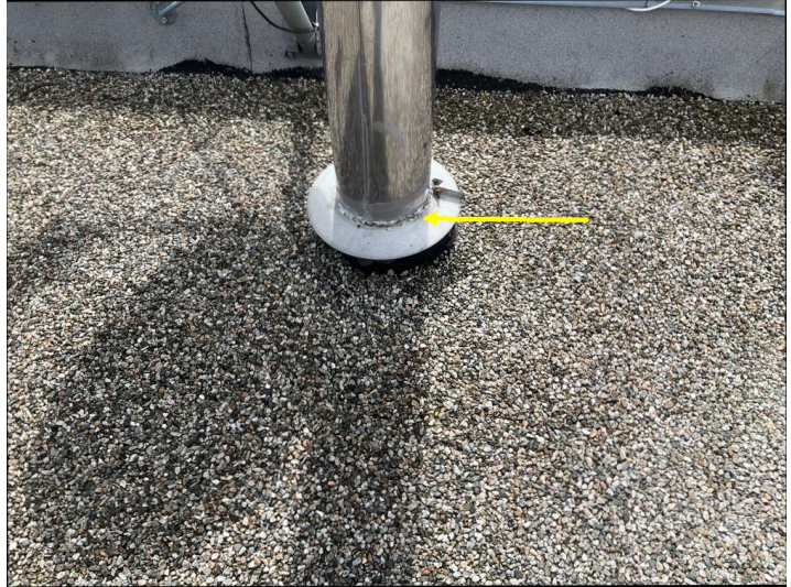
The chimney flashing is worn and should be serviced. Evidence of moisture was noted on the chimney as viewed from the living room.
