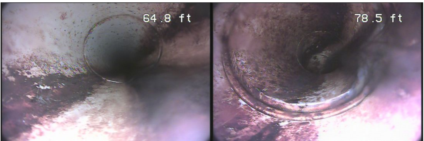
Drain waste pipe connection
