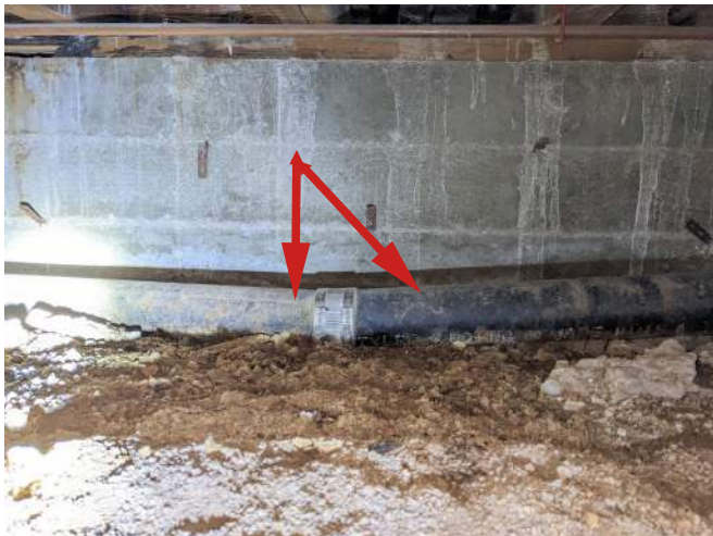
Master bathroom main drain piping not sloped correctly
