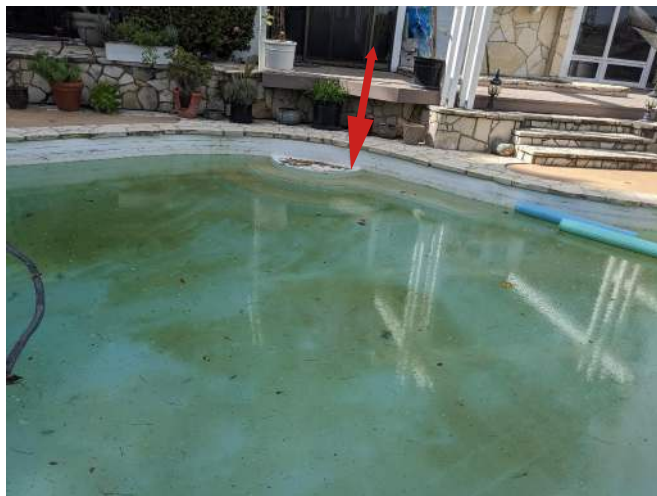
Pool water level cannot be maintained due to water leaks
