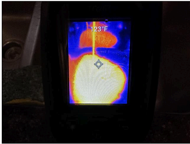
5.2 Item 1(Picture) Plumbing System
