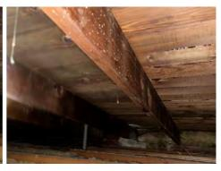
**Attic: Roof Deck Material**Solid Wood Plank, Satisfactory
