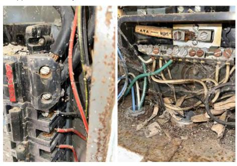
**Service Panel: Branch Circuit Wiring**Non-Metallic Shielded Copper, Satisfactory
