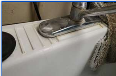
Location: LAUNDRY ROOM
