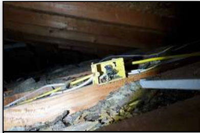
Location: CONVERTED GARAGE ACCESS
