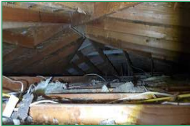
Location: CONVERTED GARAGE ACCESS
