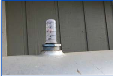
Location: LEFT EXTERIOR
