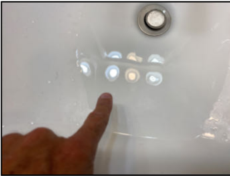
Drain operated slowly - needs to be serviced
