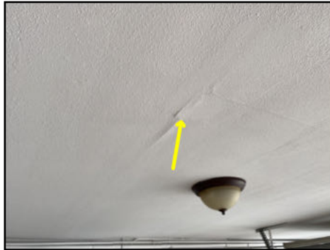
Blistered paint - cause of blistering is unknown
