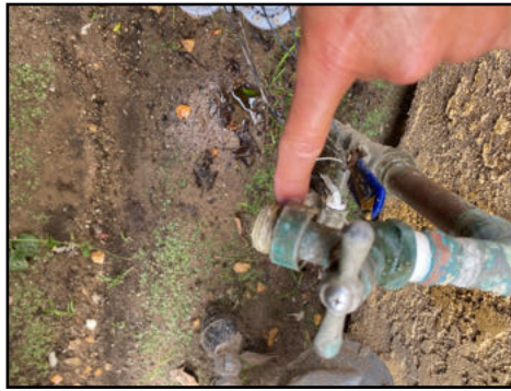
Exterior hose faucet(s) leaks/drips when turned off - needs to be serviced
