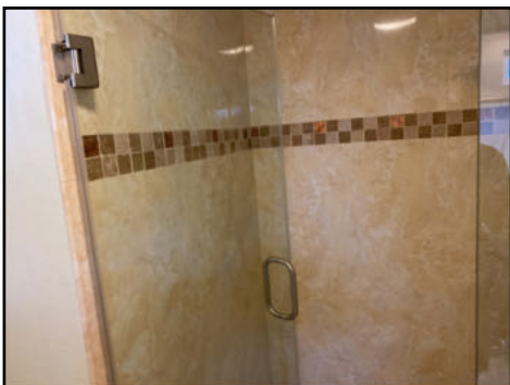
Caulking needed around perimeter
