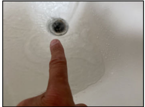
Drain stopper missing - needs to be serviced
