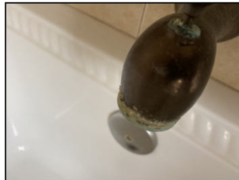
Drain stopper missing - needs to be serviced
