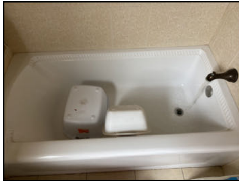
Tub fixture leaks when operated - needs to be serviced
