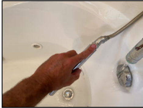
Tub fixture leaks when operated - needs to be serviced
