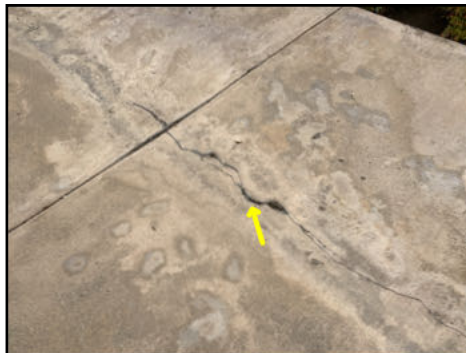
Worn with common cracks/chips - typical for age of material
