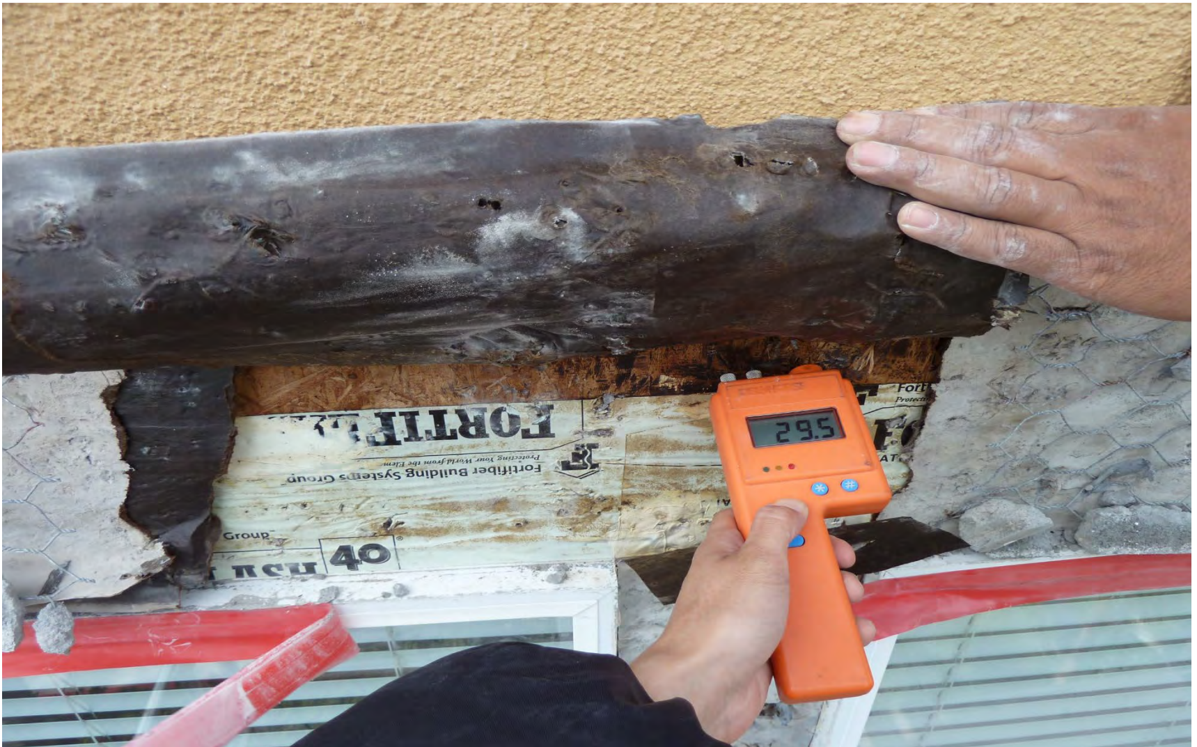
Example of water damage at windows with improper flashing
