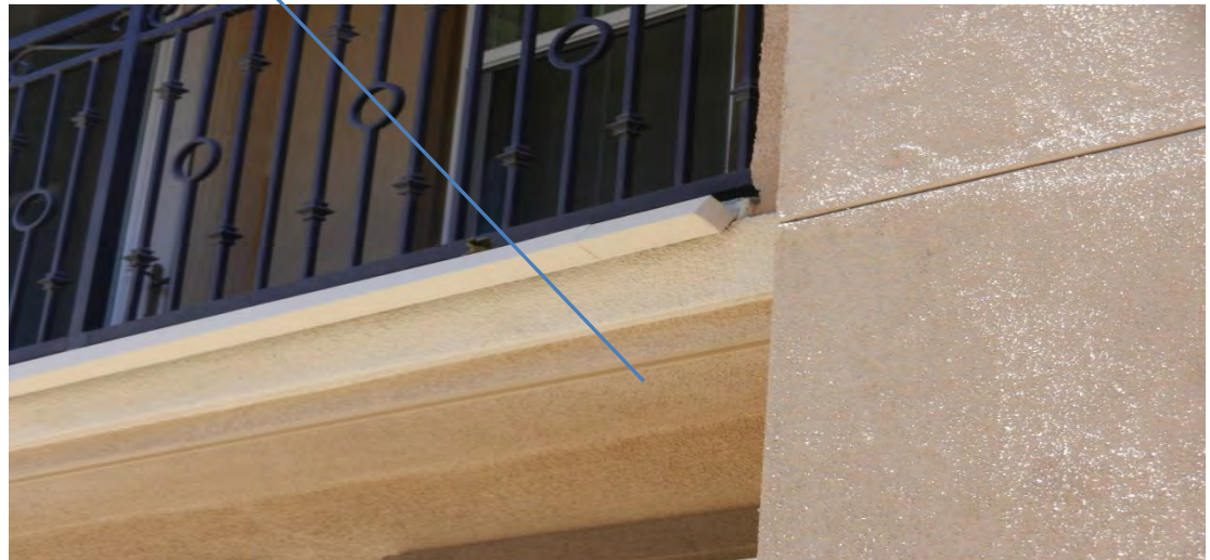
Example of water damage to deck with improper flashing and waterproofing
