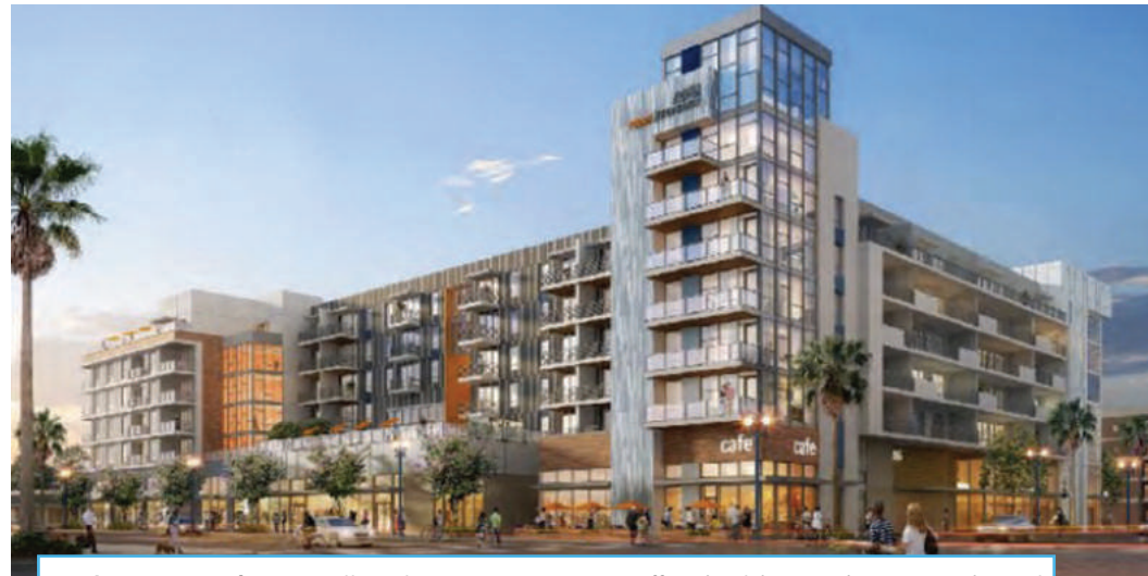
Amli Parc Broadway - will replace a government office building with 222 residential units and 8,500 square feet of retail space, including an art gallery and a "bike kitchen."
