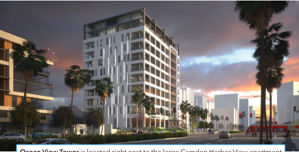
Ocean View Tower is located right next to the large Camden Harbor View apartment complex, this adaptive reuse project will transform an existing office building into a residential development with 94 apartments and 4,597 square feet of retail space.
