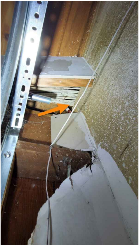
Firewall penetrations
