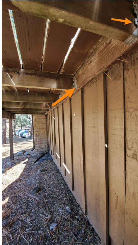
No fatteners of joists to hangers
