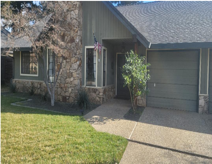
- Front of the structure.
