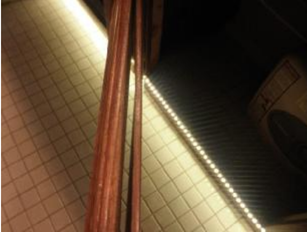
Delamination at the cabinet doors ate master bathroom vanity.
