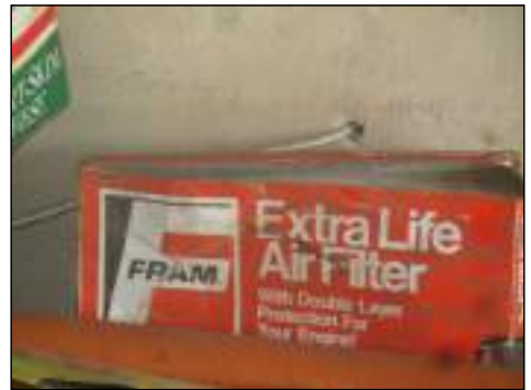
Nonmetallic sheathed wiring penetrating firewall areas - needs to be serviced to retain firewall integrity
