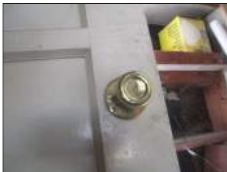
Did not lock - needs to be serviced
