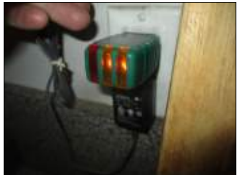
Outlets/switches had normal wear for age - no major visible defects
