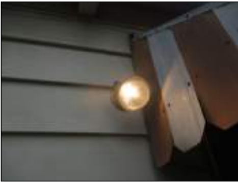
Accessible lights/switches/outlets were tested on the day of the inspection
