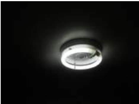
Missing/damaged outlet/switch/globe covers - recommend installation/replacement of all covers for safety
