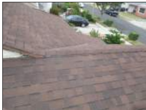
Shingles exhibited visible granule loss - normal for age of material
