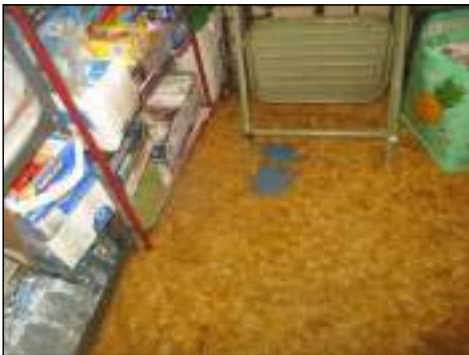
Worn/stained heavily in areas - recommend servicing
