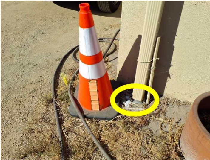
Some downspouts are missing or need to be reconnected, and should be serviced.
