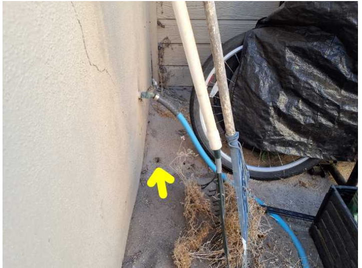
The soil is too high against the home at various areas around the residence, which should be serviced.
