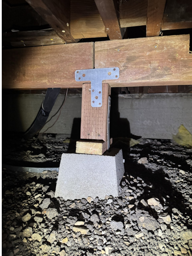
Added girder beam, and posts assembly
