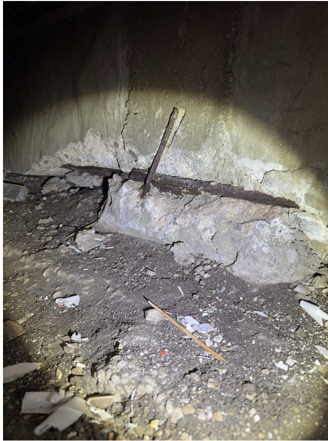
Exposed and rusted rebar
