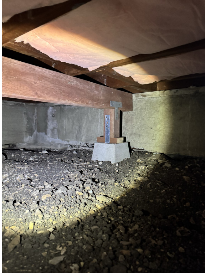
New girder beam and pier assembly
