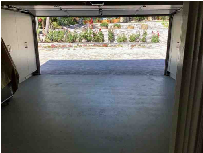
2-Car Attached Garage
