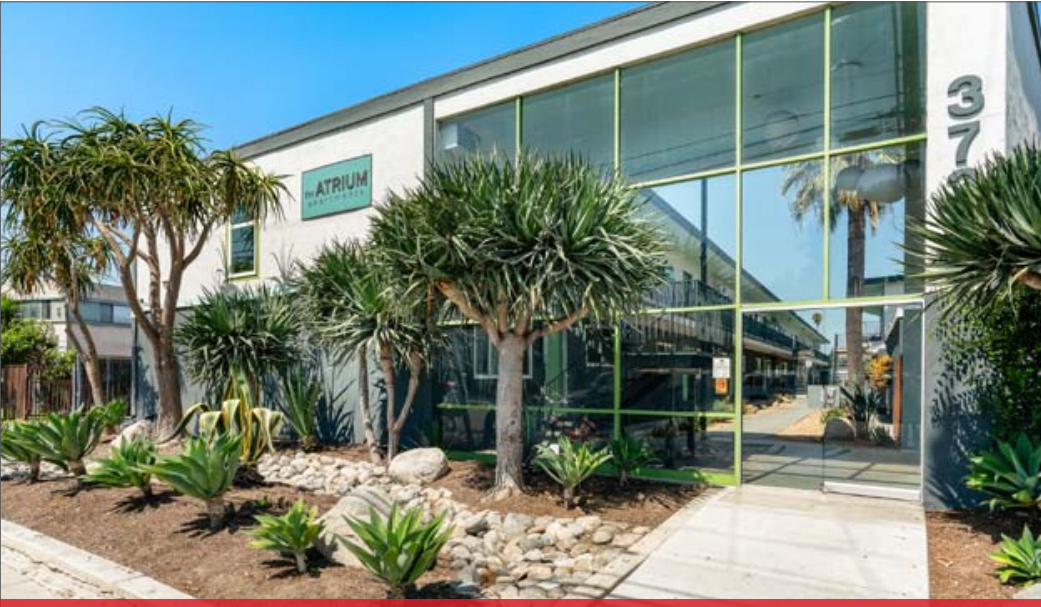
Fully upgraded and turnkey 39-unit community
