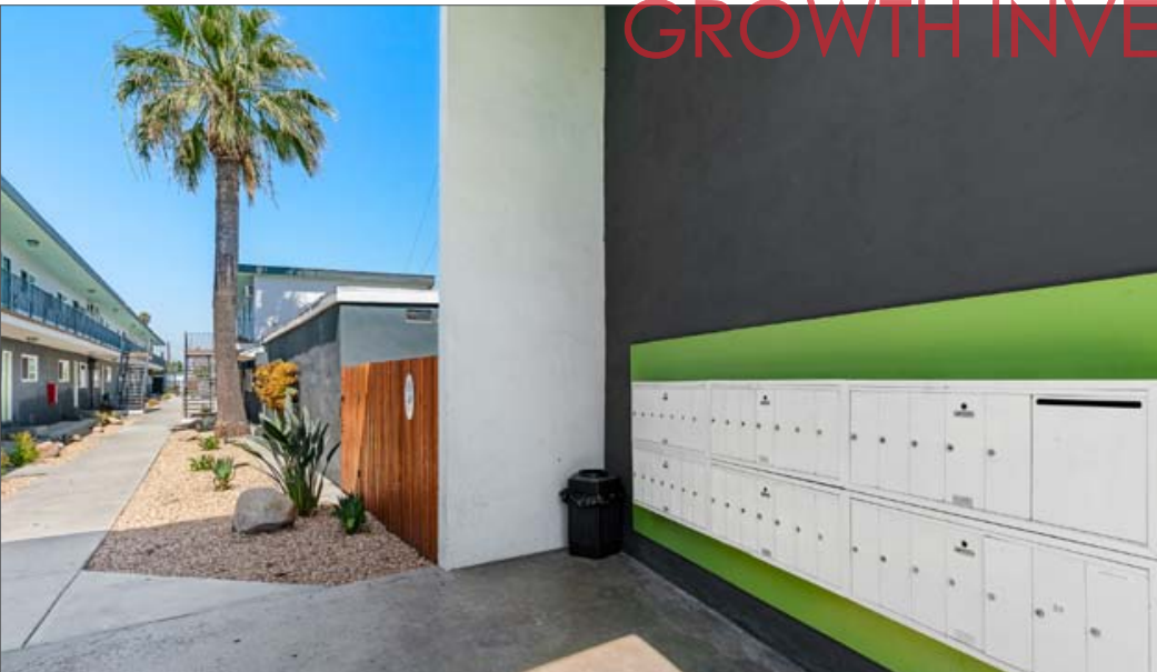
BRAND NEW Mailboxes and an atrium entrance
