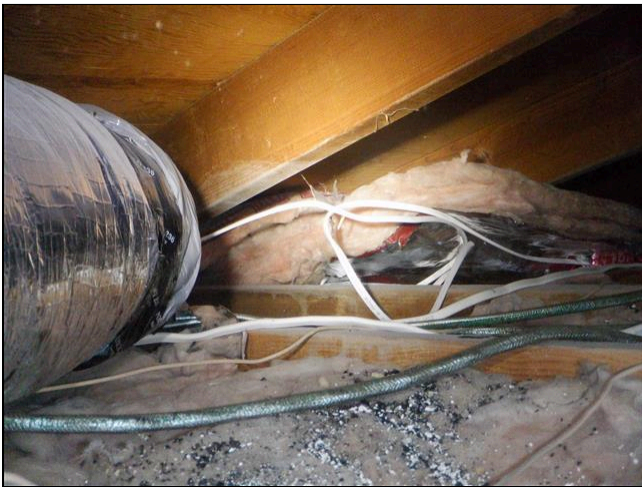
1.5 Item 5(Picture) Attic Insulation
