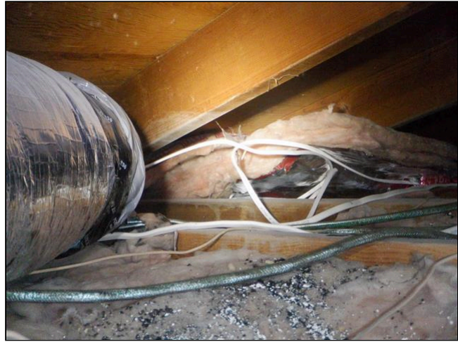
1.4 Item 6(Picture) Roof Framing/Roof Decking
