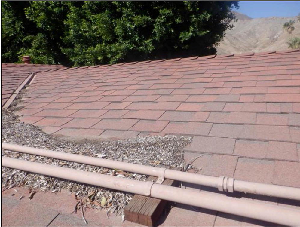
1.0 Item 3(Picture) Roof Covering
