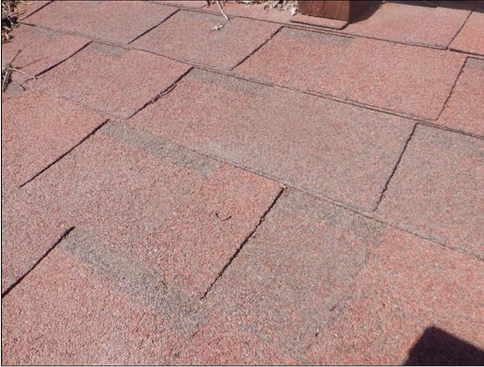
1.0 Item 5(Picture) Roof Covering
