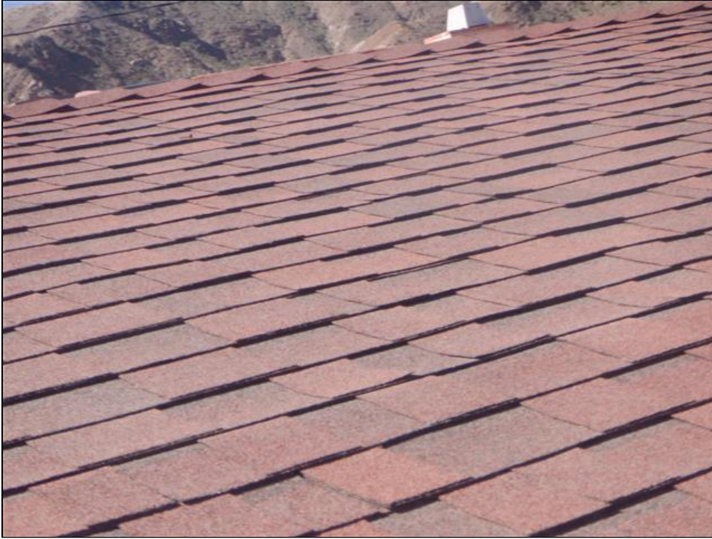
1.0 Item 7(Picture) Roof Covering
