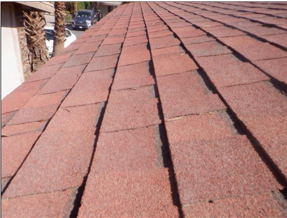
1.0 Item 14(Picture) Roof Covering
