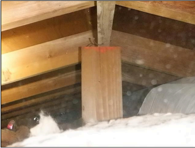
1.4 Item 5(Picture) Roof Framing/Roof Decking
