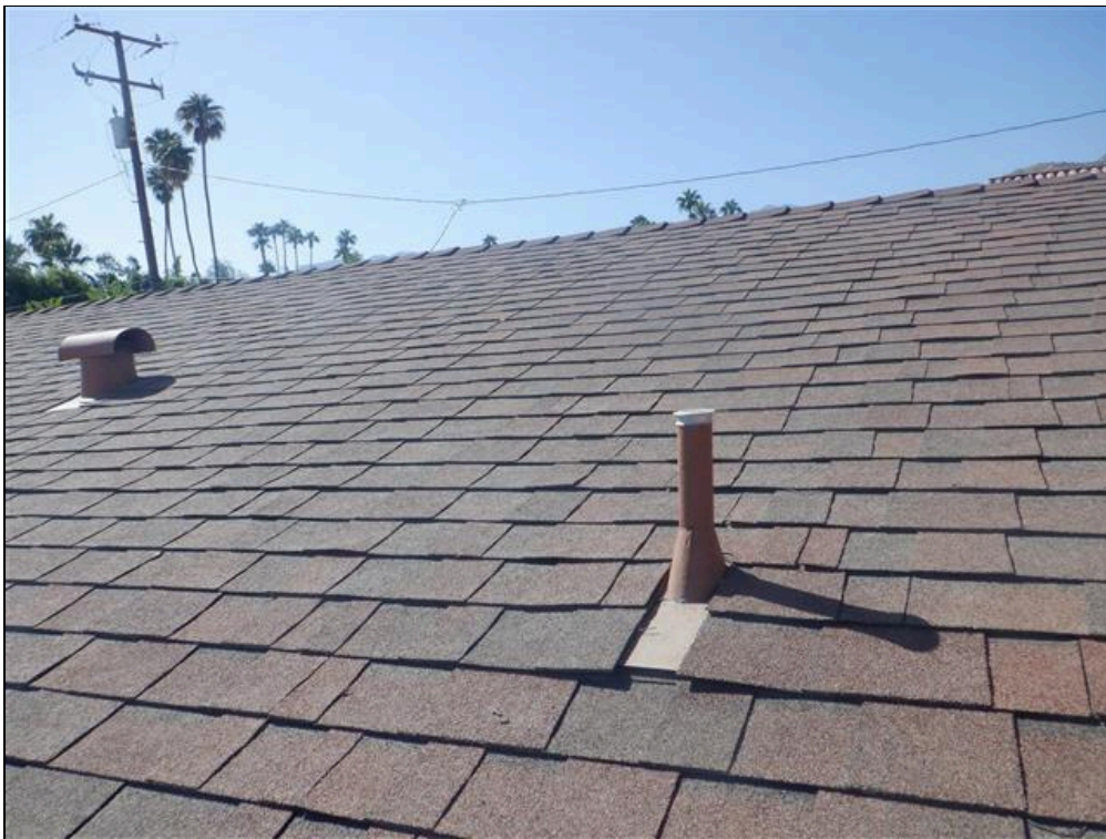
1.0 Item 4(Picture) Roof Covering
