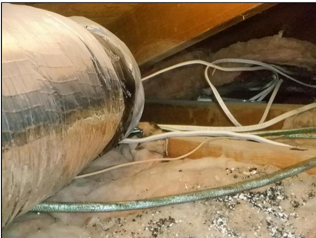
1.5 Item 1(Picture) Attic Insulation
