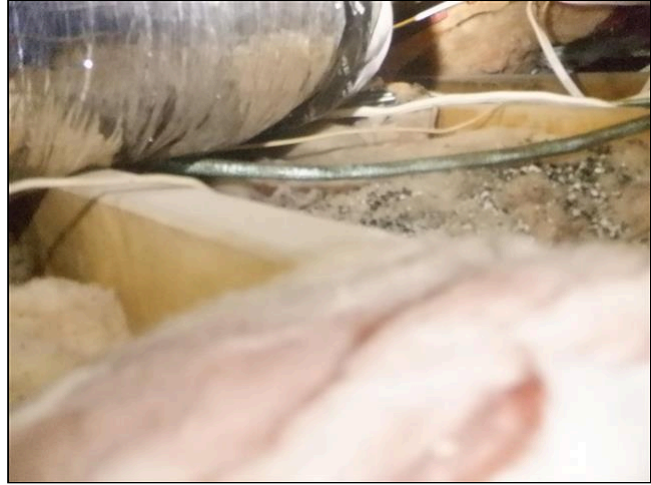
1.5 Item 4(Picture) Attic Insulation
