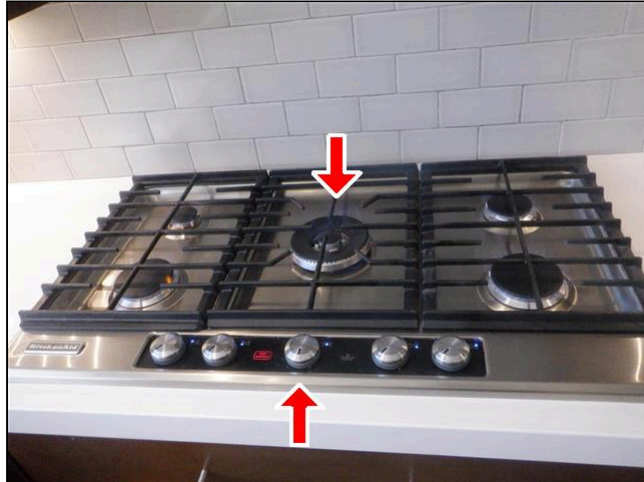
4.9 Item 1(Picture) Center Burner/Igniter
