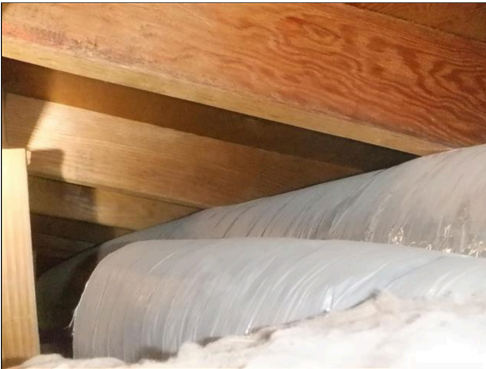
1.4 Item 4(Picture) Roof Framing/Roof Decking
