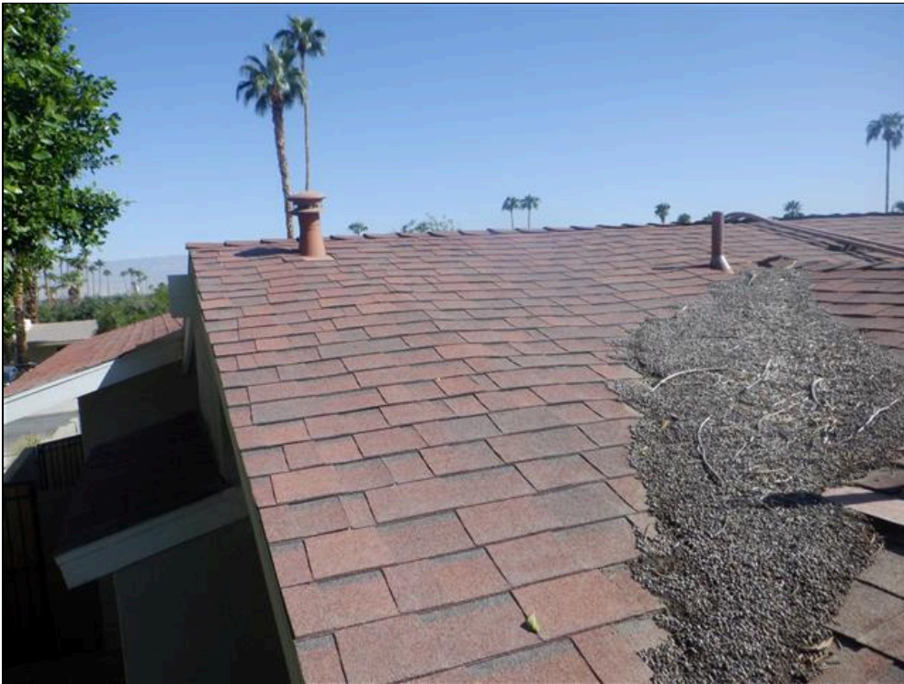
1.0 Item 12(Picture) Roof Covering
