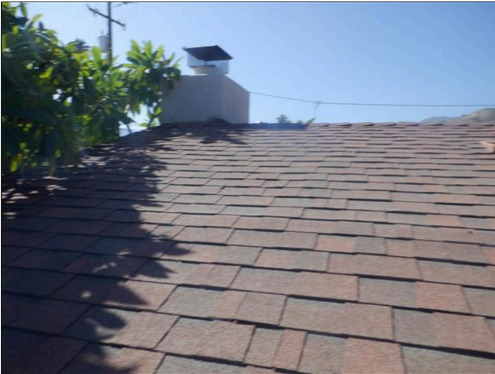
1.0 Item 6(Picture) Roof Covering
