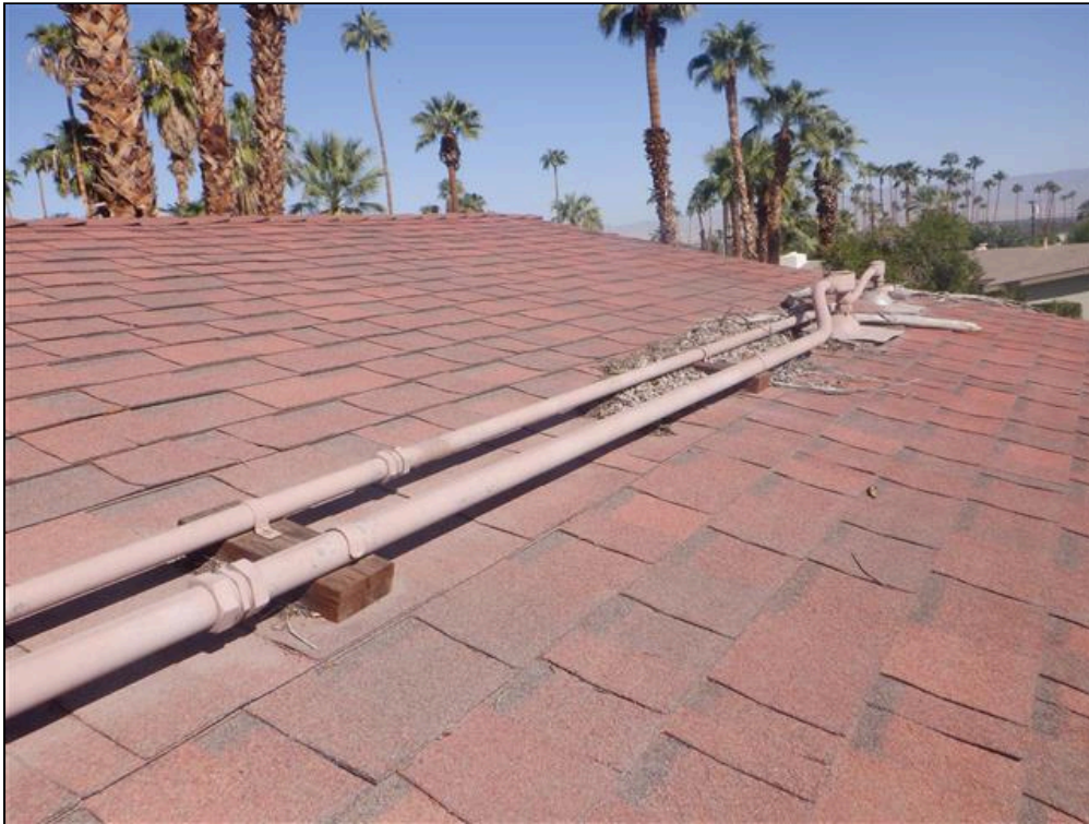
1.0 Item 1(Picture) Roof Covering
