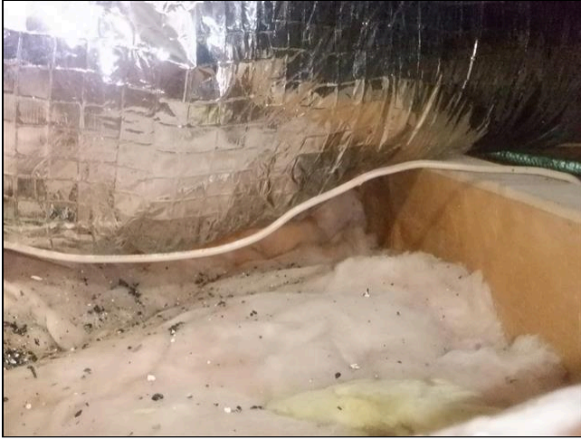
1.5 Item 3(Picture) Attic Insulation
