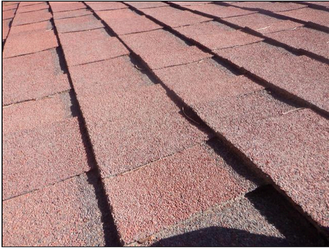
1.0 Item 15(Picture) Roof Covering
