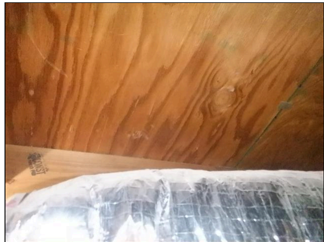
1.4 Item 2(Picture) Roof Framing/Roof Decking
