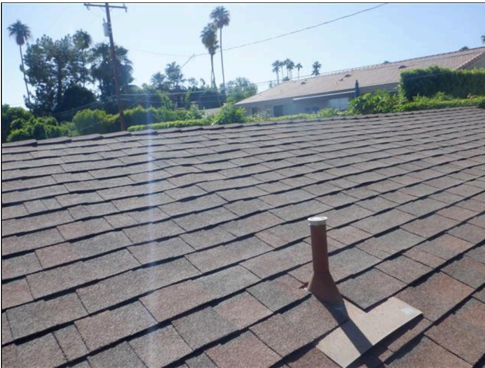
1.0 Item 10(Picture) Roof Covering
