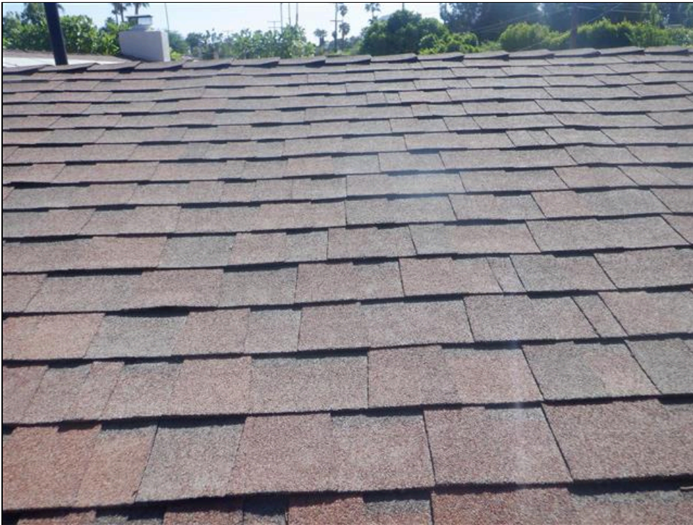
1.0 Item 8(Picture) Roof Covering
