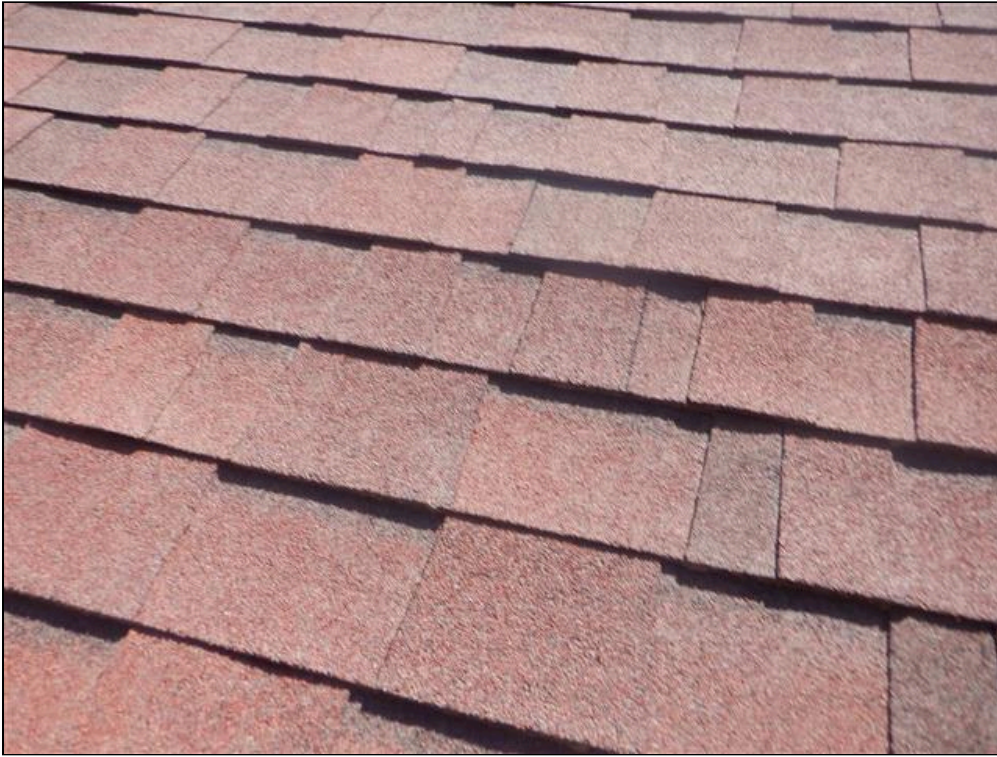
1.0 Item 11(Picture) Roof Covering
