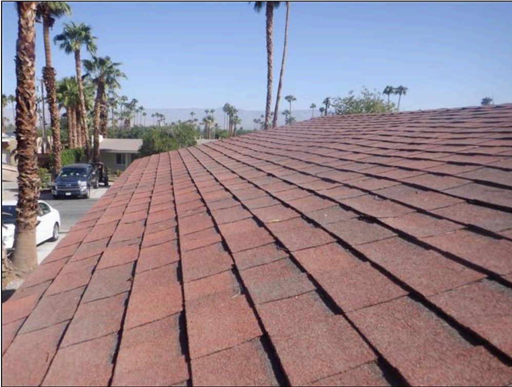
1.0 Item 13(Picture) Roof Covering
