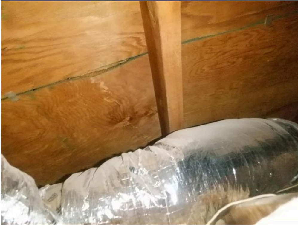
1.4 Item 3(Picture) Roof Framing/Roof Decking
