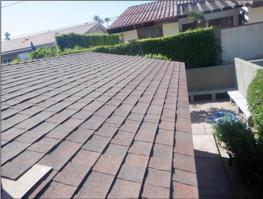
1.0 Item 9(Picture) Roof Covering
