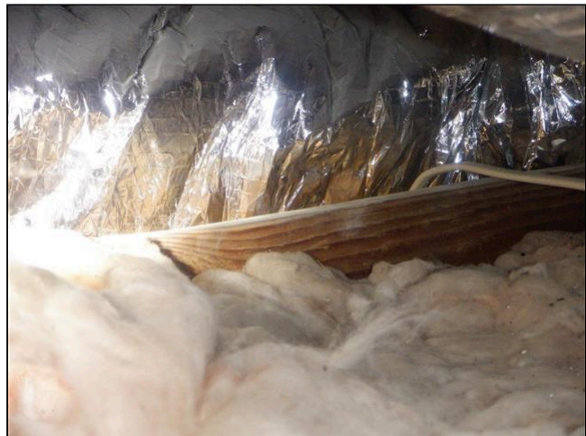
1.5 Item 2(Picture) Attic Insulation
