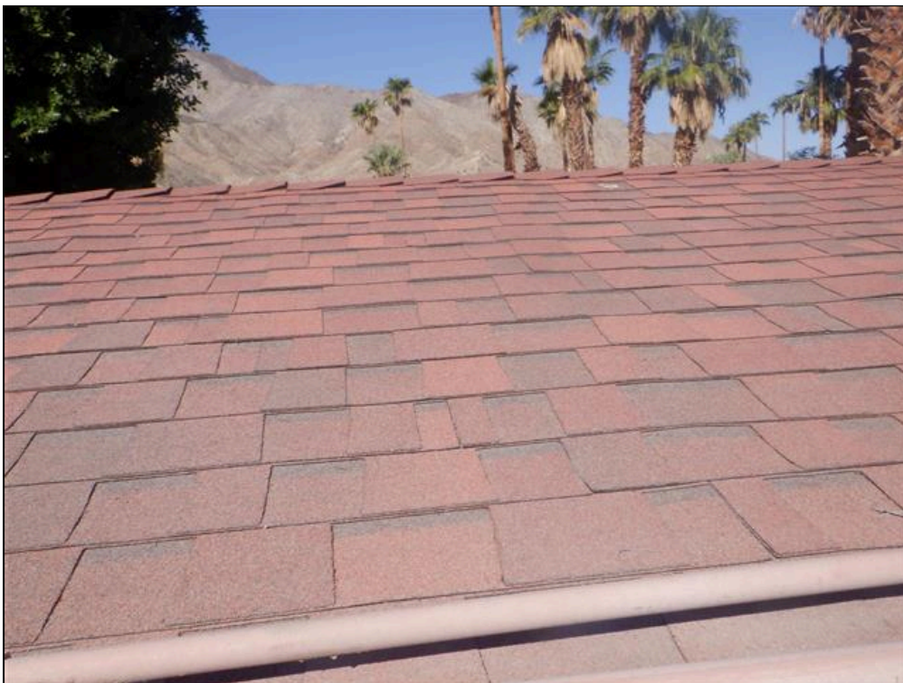
1.0 Item 2(Picture) Roof Covering
