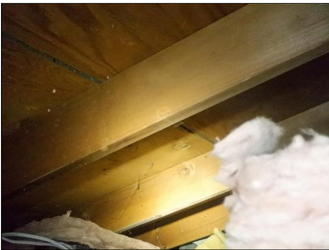
1.4 Item 7(Picture) Roof Framing/Roof Decking
