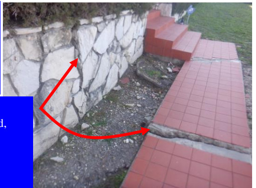
...and some replaced flashings indicate past issues
