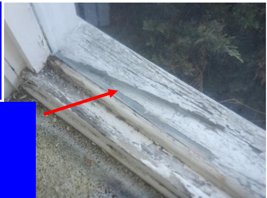
...throughout the eaves...
