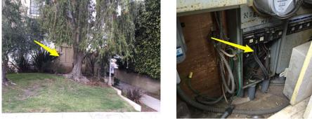
**CR** The circuit breakers were not labeled. We recommend they be accurately labeled to allow individual circuits to be shut off for maintenance or emergency needs.
