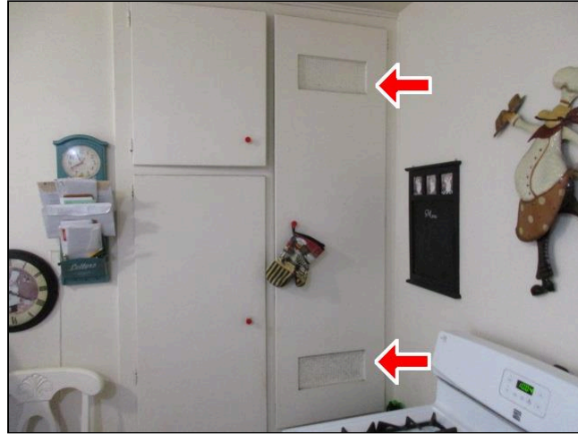
Vents Covered, Typical
