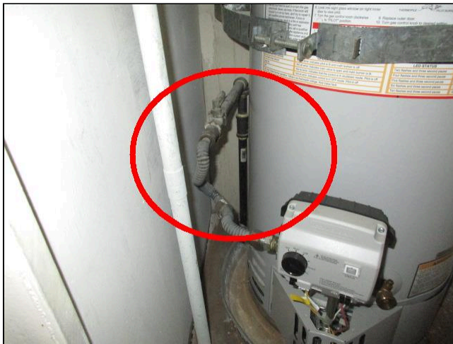
Add Sediment Traps, Water Heaters, Typical
