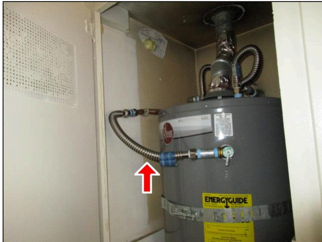
Piping Incorrectly Installed Upward, Unit C
