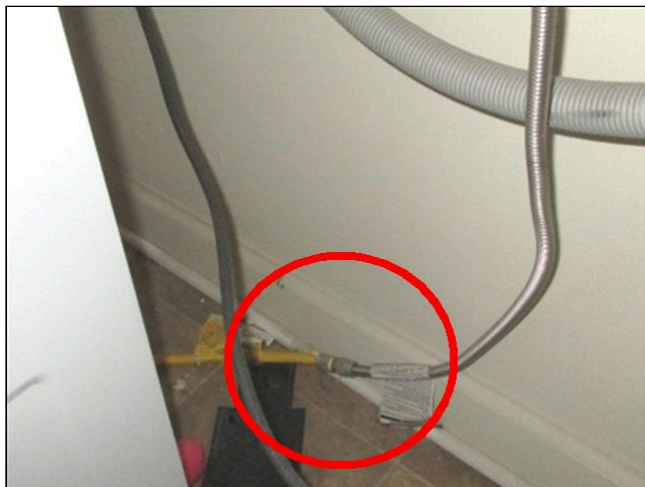
Flex Connectors Joined Together
