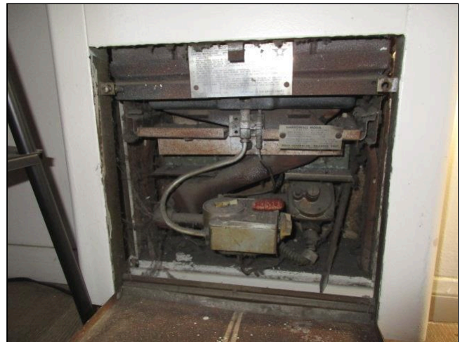
Add Sediment Traps, Wall Furnaces, Typical
