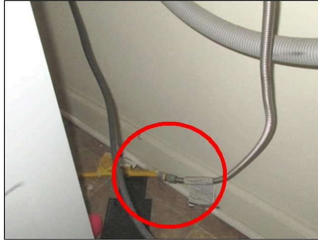
Flex Connectors Joined Together
