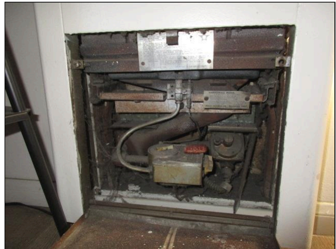
Add Sediment Traps, Wall Furnaces, Typical
