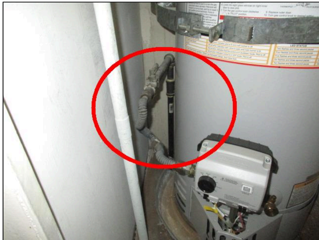
Add Sediment Traps, Water Heaters, Typical
