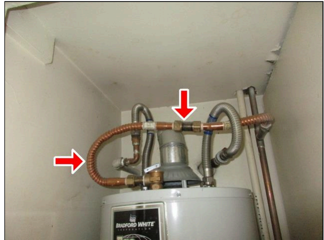
Piping Incorrectly Installed Upward, Unit A
