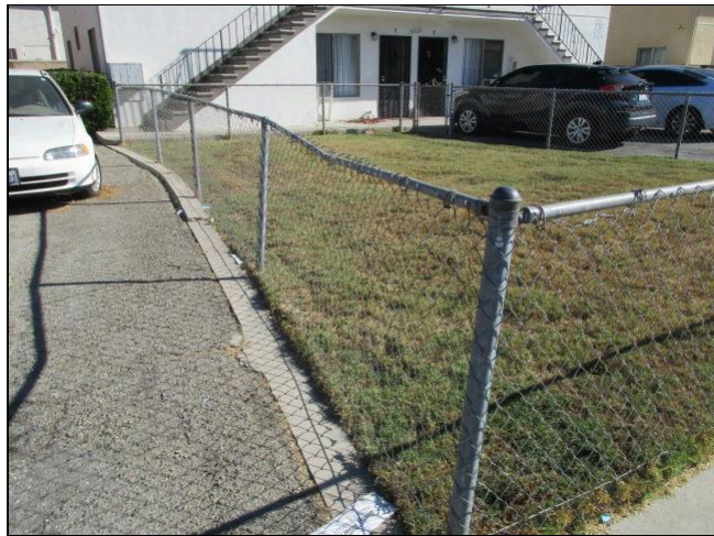
Damaged Chainlink
