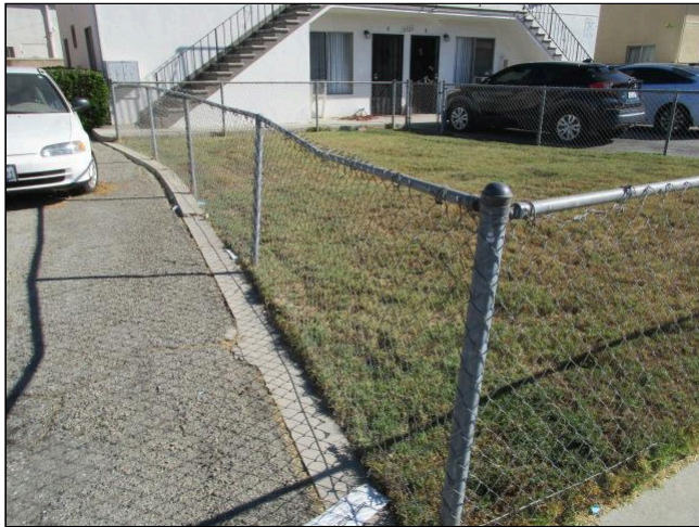
Damaged Chainlink
