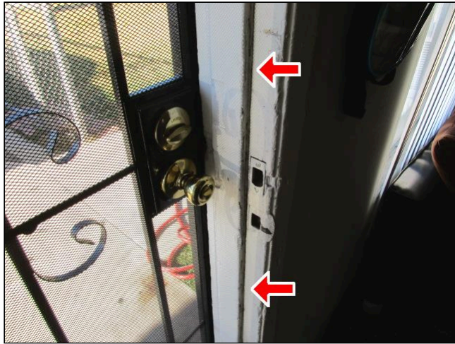
Add Weather Stripping
