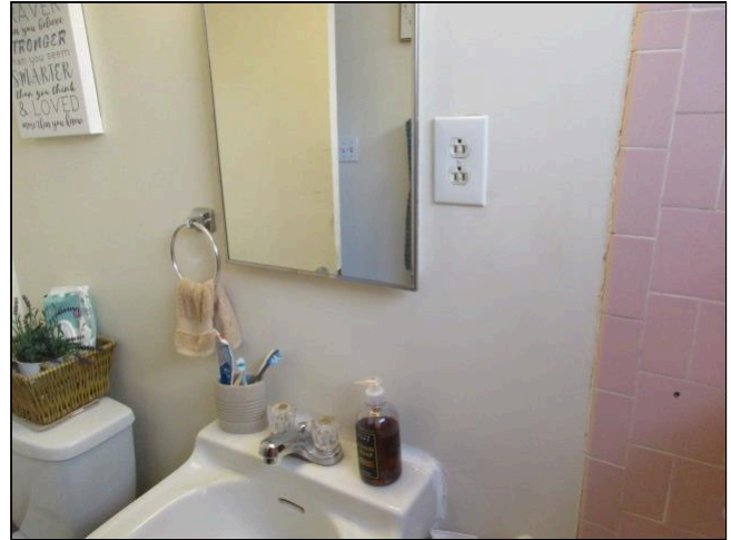
Add Bathroom GFCI's
