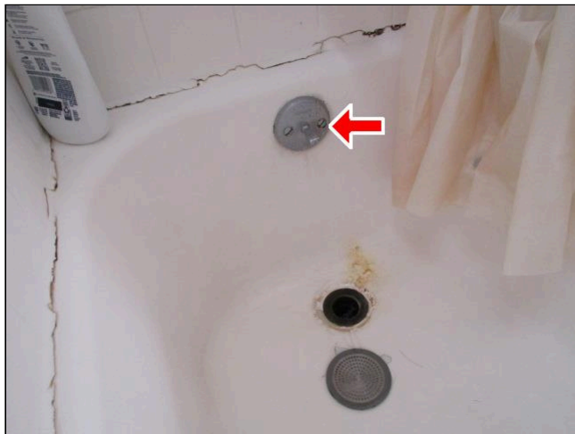
Stopper Not Operational, Unit D
