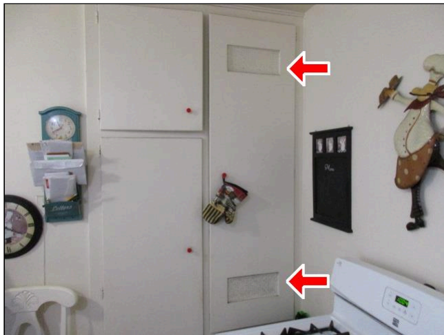
Vents Covered, Typical
