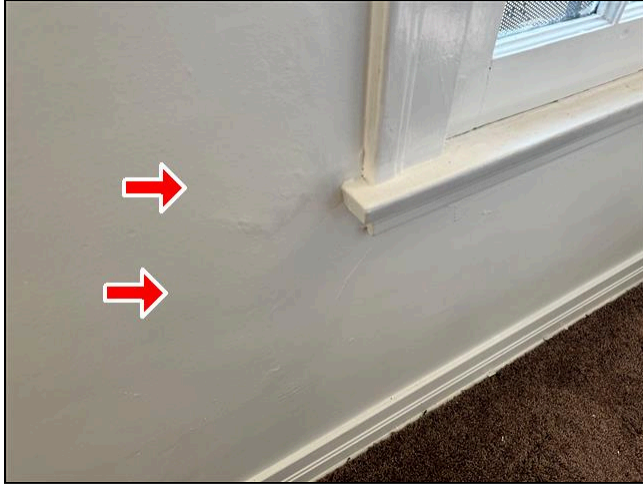
8.1 Item 1 (Picture) Interiors
