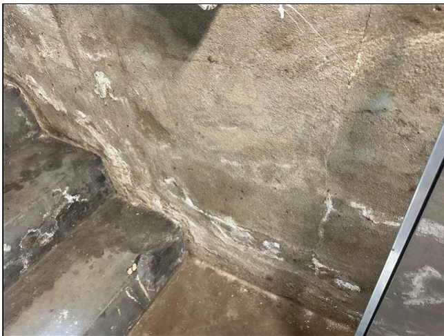
Item 13 - Item 1 (Picture) Structural Components
