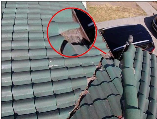
1.0 Item 5 (Picture) Roofing
