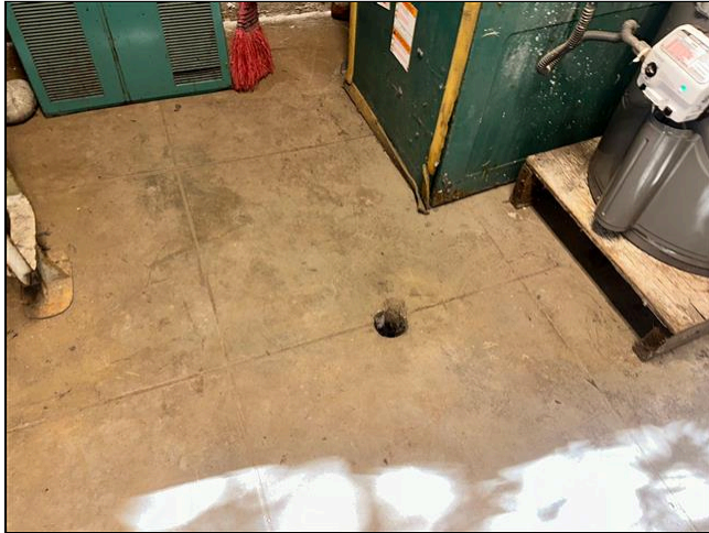
3.0 Item 6 (Picture) Structural Components
