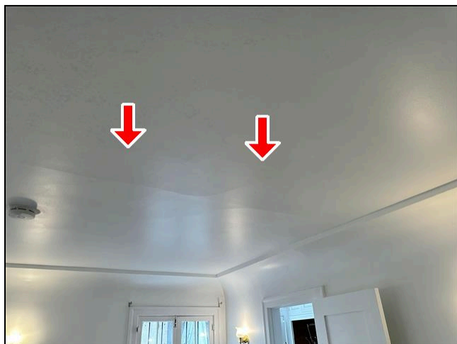
8.1 Item 2 (Picture) Interiors
