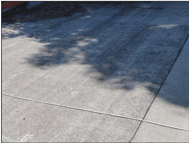
1.0 Item 3 (Picture) Roofing
