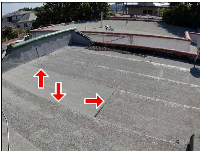
1.0 Item 1 (Picture) Roofing
