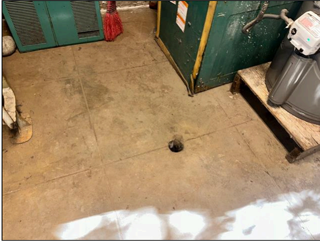
Item 14 - Item 1 (Picture) Structural Components
