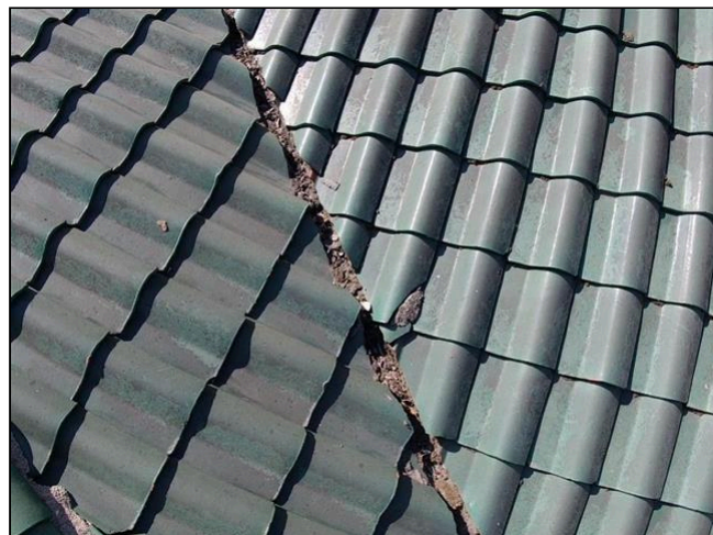
Item 4 - Item 2 (Picture) Roofing
