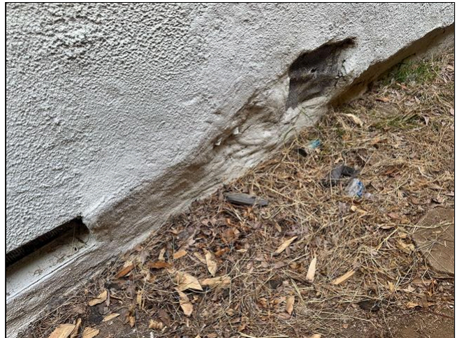
3.0 Item 2 (Picture) Structural Components
