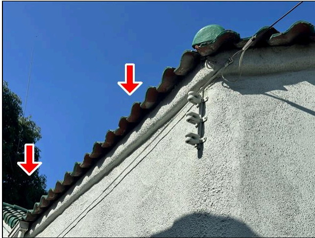
1.0 Item 7 (Picture) Roofing
