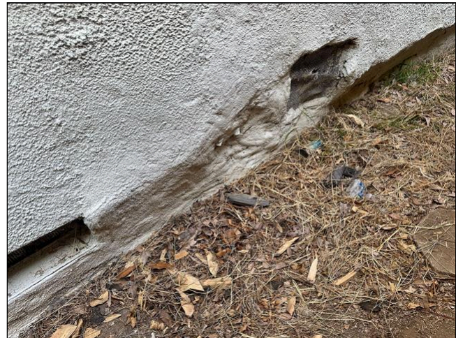
Item 10 - Item 2 (Picture) Structural Components
