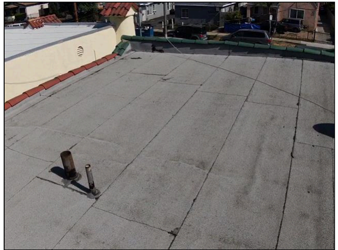
1.0 Item 4 (Picture) Roofing
