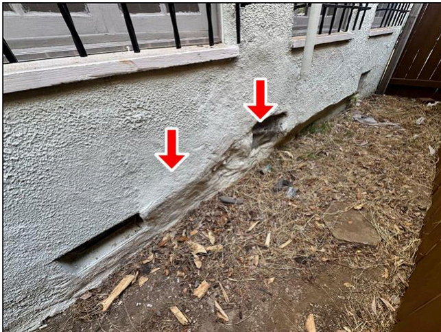
Item 10 - Item 1 (Picture) Structural Components
