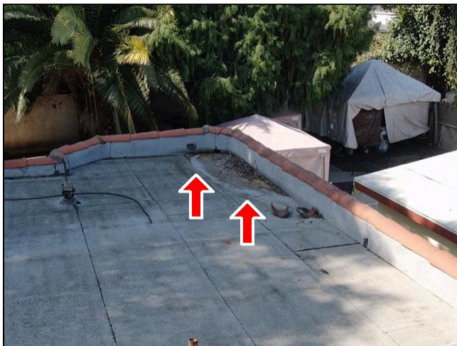
1.3 Item 1 (Picture) Roofing
