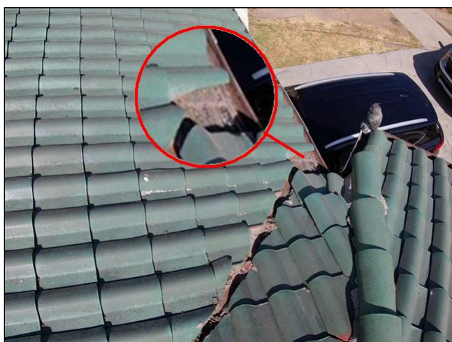
Item 2 - Item 1 (Picture) Roofing
