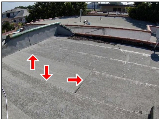
Item 1 - Item 1 (Picture) Roofing
