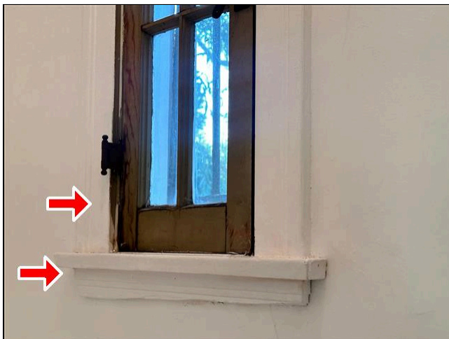
8.3 Item 2 (Picture) Interiors
