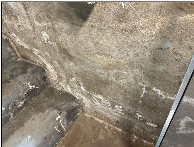
3.0 Item 4 (Picture) Structural Components
