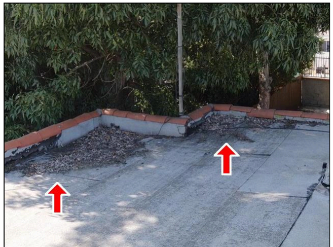
1.3 Item 2 (Picture) Roofing
