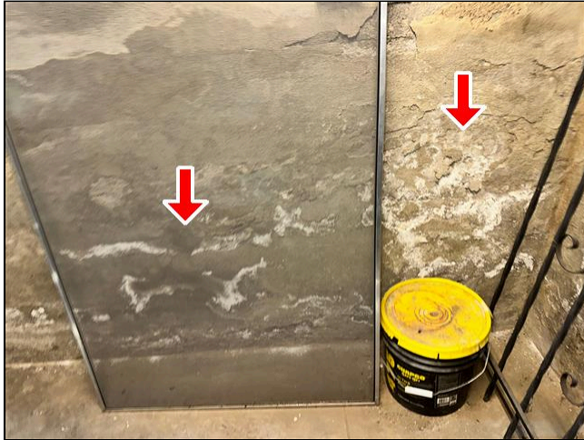
3.0 Item 3 (Picture) Structural Components
