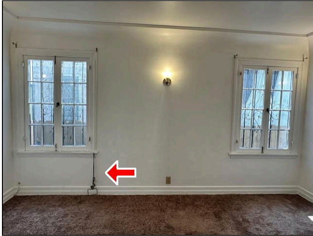
8.3 Item 1 (Picture) Interiors
