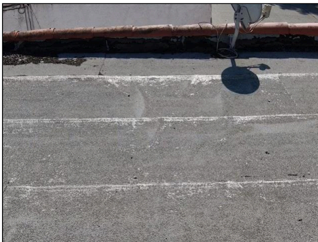
Item 1 - Item 2 (Picture) Roofing
