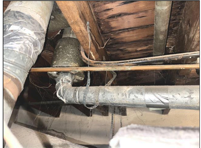
3.2 Item 2 (Picture) Structural Components
