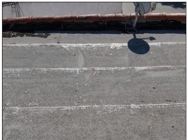
1.0 Item 2 (Picture) Roofing
