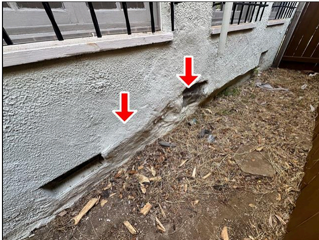
3.0 Item 1 (Picture) Structural Components
