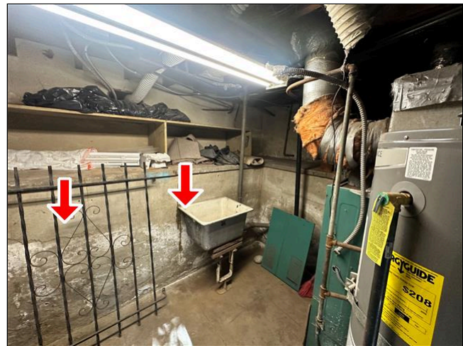
Item 13 - Item 2 (Picture) Structural Components
