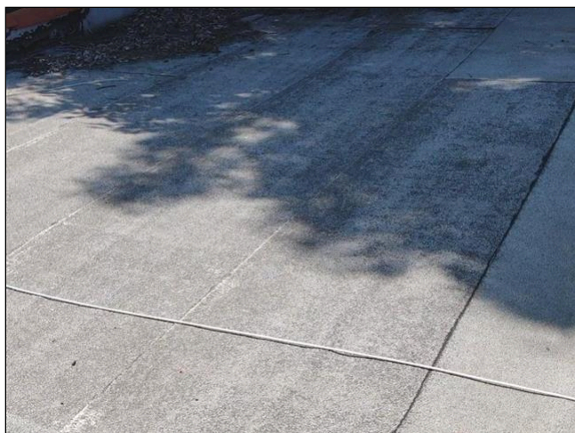
Item 1 - Item 3 (Picture) Roofing
