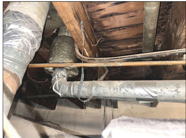
Item 15 - Item 2 (Picture) Structural Components
