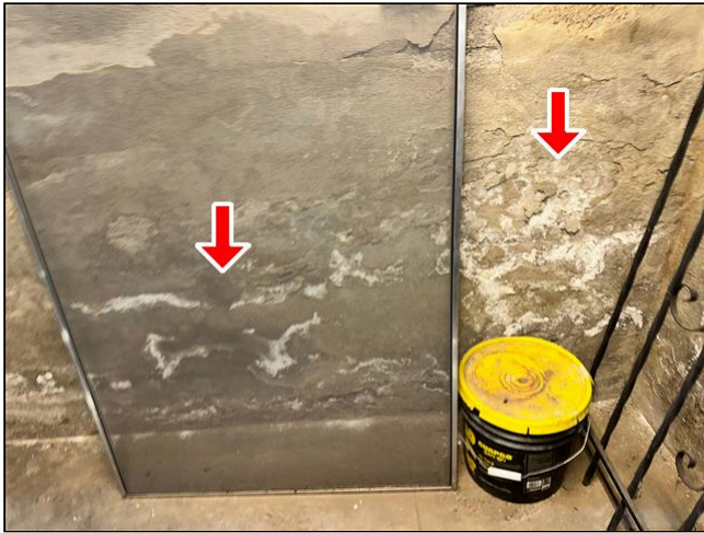
Item 12 - Item 1 (Picture) Structural Components
