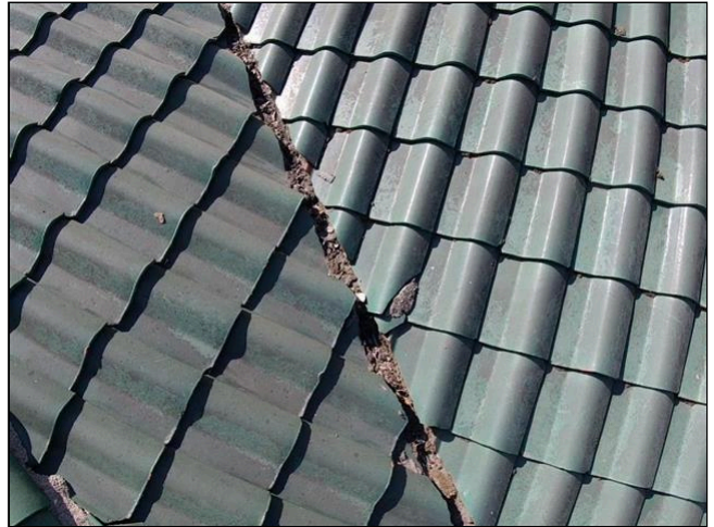
1.0 Item 8 (Picture) Roofing
