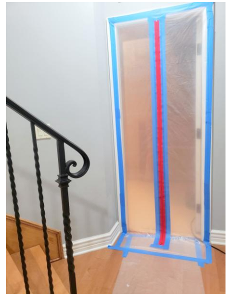
35. Closet's sealed door
