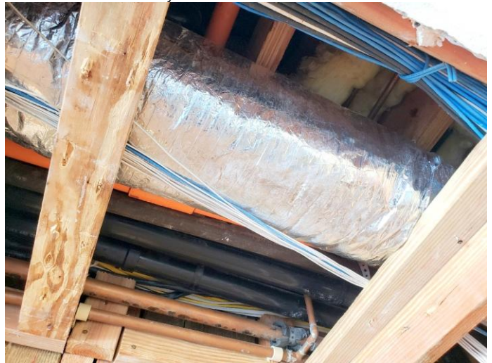
4. Portion of the in-ceiling lumber after cleaning
