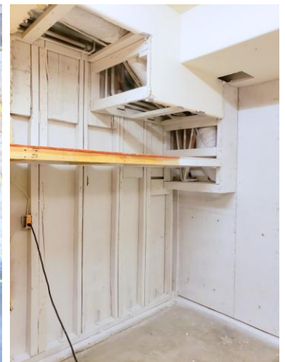
12. South-east corner after encapsulation
