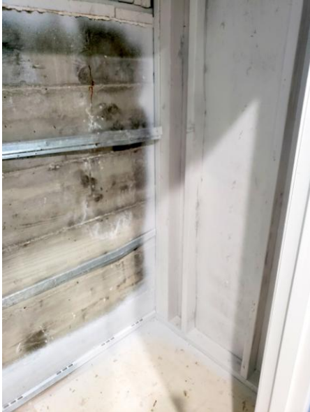
25. Closet after encapsulation
