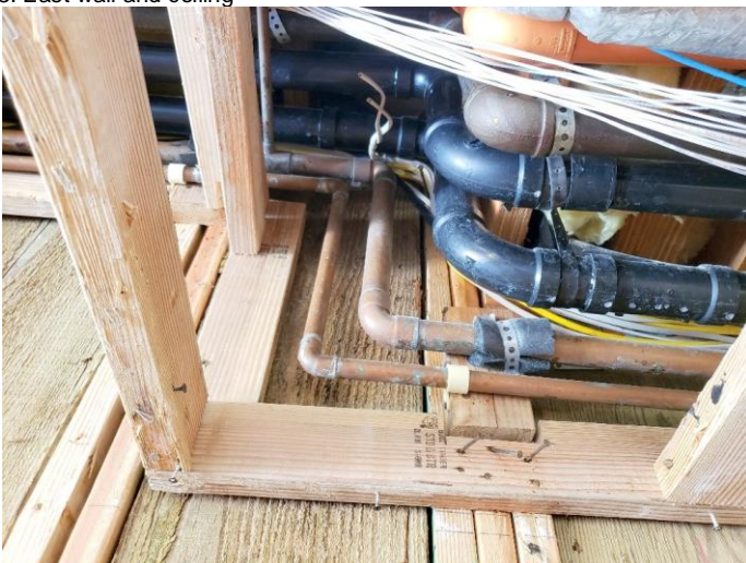
5. Portion of the in-wall and in-ceiling lumber after cleaning and chem. treatments.
