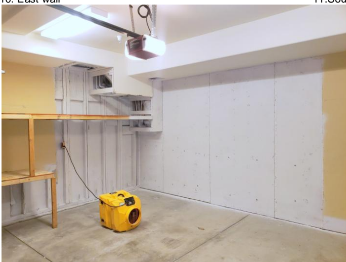
13. South and east walls after encapsulation
