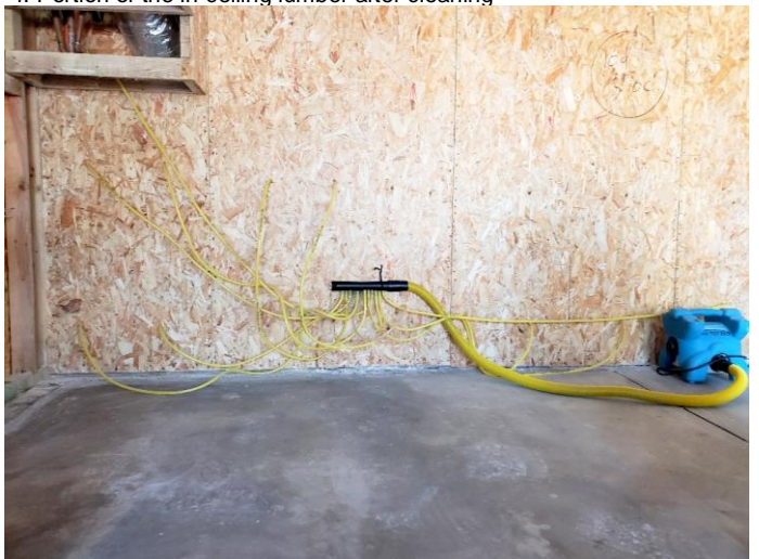
6. South wall after cleaning and chem. treatments. In-wall drying system installed
