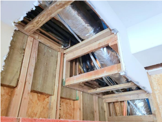
3. East wall and ceiling
