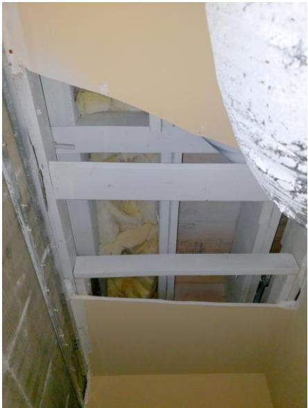
33. Ceiling after encapsulation
