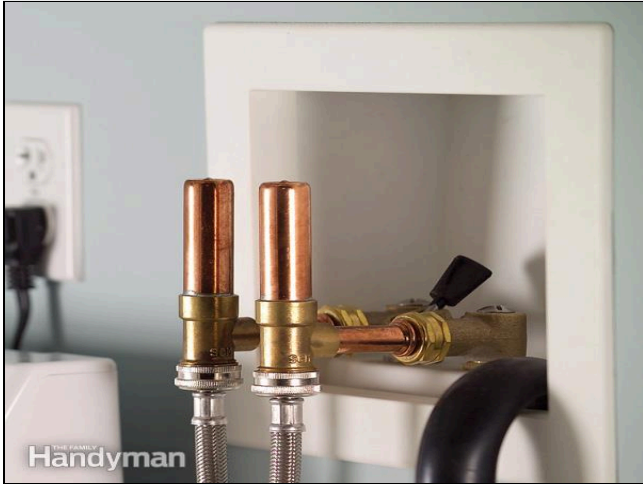
6.3 Item 1 (Picture) HV
