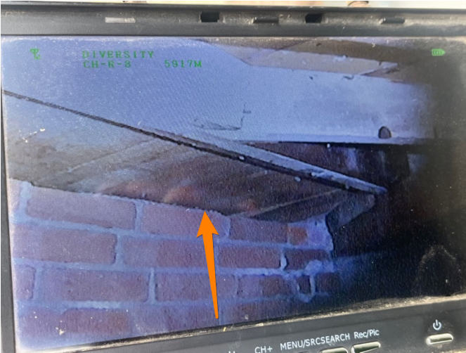
Wood form boards under hearth extension
