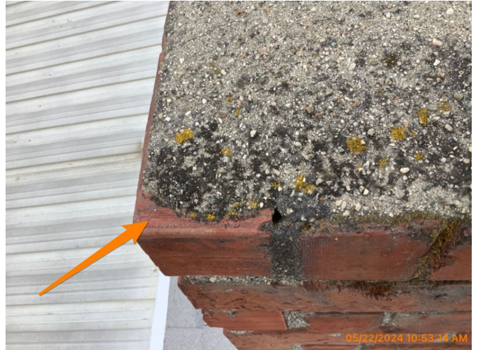
Crown does not extend to the edges
