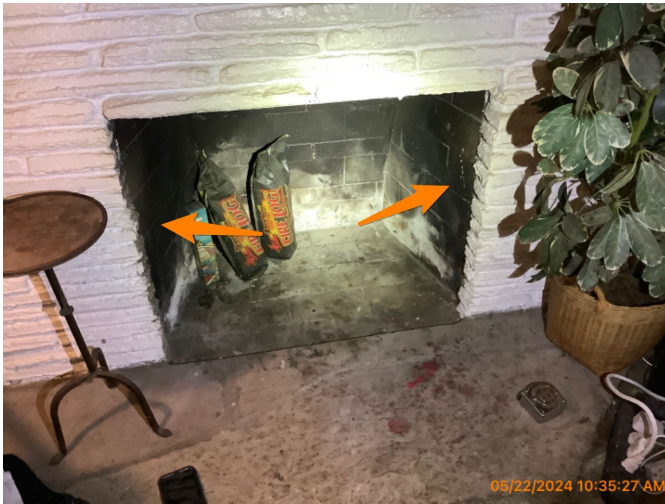
Approximate location of surround gaps
