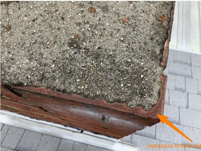
Crown does not extend to the edges
