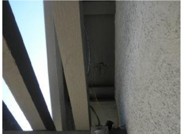
Evidence of a leak with moisture damage to the plywood at the gable above the exterior door.
