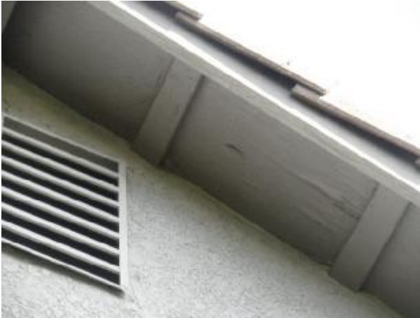
Evidence of a leak with moisture damage to the plywood at the west facing gable.
