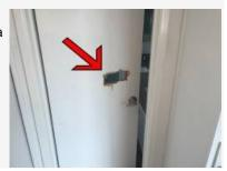
Bi-fold closet door is stuck, therefore does not open at the left rear bedroom. We recommend correction using appropriate methods by a qualified door specialist.
