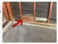
The diameter of the vent screen mesh is too large. The condition is conducive to insect / vermin intrusion into the building. Replacement with an appropriate screening material is recommended.
