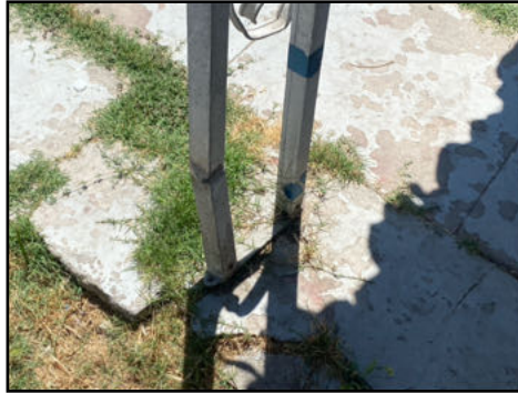
Post base dented/buckling - needs to be serviced
