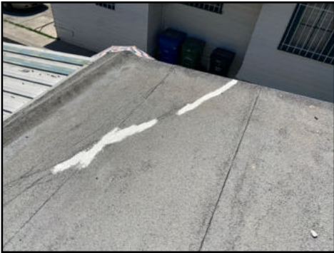
Patching observed in areas on roof materials - inspector is unable to guarantee the adequacy of these repairs - recommend maintaining a continuous water tight seal in these areas
