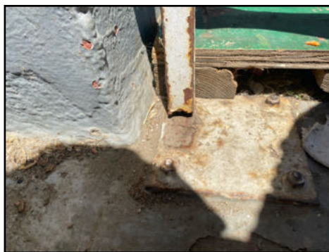
Loose rails - unsafe - needs to be serviced
