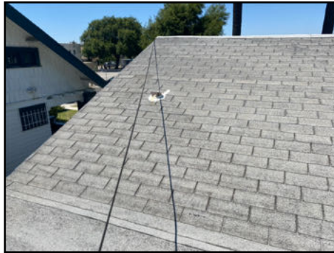
Patching observed in areas on roof materials - inspector is unable to guarantee the adequacy of these repairs - recommend maintaining a continuous water tight seal in these areas
