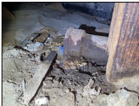
Leak found under toilet - needs to be serviced
