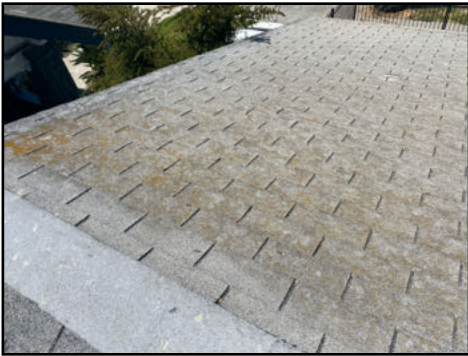
Moss growth present in areas - sign of moisture accumulation and lack of sunlight for drying - recommend servicing as part of seasonal maintenance
