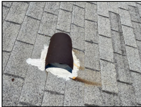
Re-roof covers flashings - irregular installation - needs further evaluation by a licensed roofer
