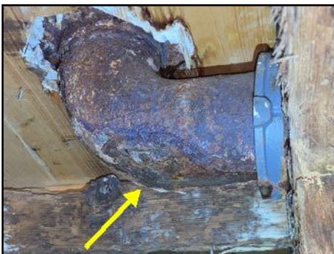
Leak found under toilet - needs to be serviced
