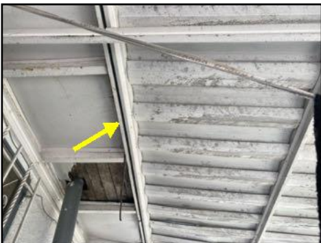
Structure attached to fascia board – irregular installation – recommend licensed contractor to evaluate
