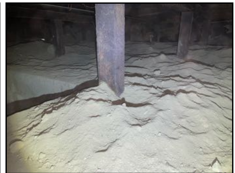
Posts in contact with soil - needs to be serviced - consult the termite report
