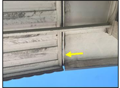
Structure attached to fascia board – irregular installation – recommend licensed contractor to evaluate
