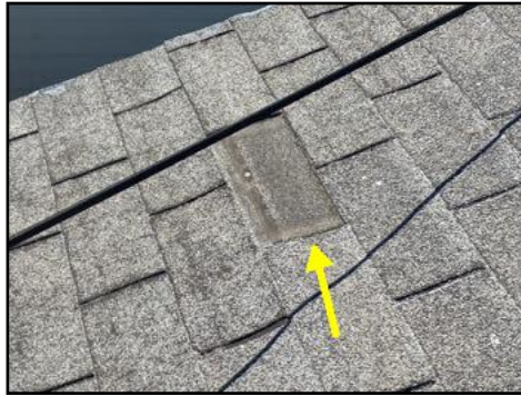
Missing/damaged shingles/tiles in areas - needs to be serviced
