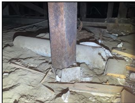
Posts in contact with soil - needs to be serviced - consult the termite report
