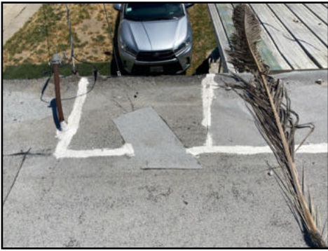
Patching observed in areas on roof materials - inspector is unable to guarantee the adequacy of these repairs - recommend maintaining a continuous water tight seal in these areas
