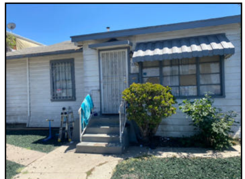
Structure attached to fascia board – irregular installation – recommend licensed contractor to evaluate
