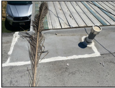
Patching observed in areas on roof materials - inspector is unable to guarantee the adequacy of these repairs - recommend maintaining a continuous water tight seal in these areas
