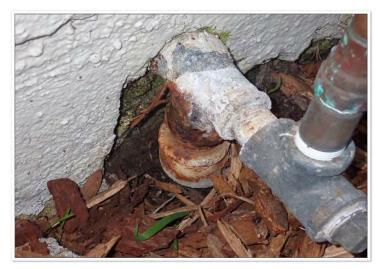
Since main shut-off valves are operated infrequently, it is not unusual for them to become frozen over time. They often leak or break when operated after a period of inactivity. For this reason main shut-off valves are not tested during a home inspection. We suggest caution when operating shut-offs that have not been turned for a long period of time. All shut-off valves and angle stops should be turned regularly to ensure free movement in case of emergency.
