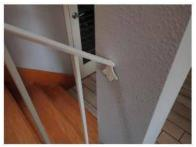
Safety Concern: The handrail was loose (not properly secured). This condition is a safety hazard.
