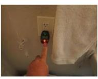
Corrections Recommended: An ungrounded three-prong receptacle was observed at master bathroom. We recommend that any ungrounded three-prong receptacle be grounded.
