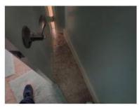
Corrections Recommended: One or more door stops were missing. This condition will likely lead to damage to the wall surfaces. Repair as needed.
