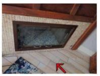
Safety Concern: The height of fireplace hearth extension was not distinguishable from the surrounding flooring. The hearth extension is a designated space where combustible materials should not be located. Repair as needed for safety.
