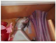
Corrections Recommended: The exhaust vent pipe was reduced to a smaller diameter. Repair as needed for proper operation.
