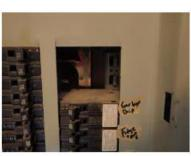
Safety Concern: The dead-front cover to electric sub panel in the laundry room was missing twist-outs/knock-outs at unused breaker slots. All openings in the cover should be filled/closed to minimize access by insects, rodents or unauthorized personnel.
