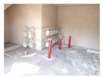
The gas meter and or shut off was located at the rear of the building. The main gas supply shut-off valve was located on the riser pipe between the ground and the meter.
