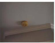
Further Evaluation: The smoke alarms appear to be older the 10 years. Aging smoke alarms don't operated as efficiently and often are the source for nuisance alarms The industry standards recommends replacing older smoke alarms. Repair as needed.
