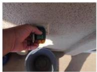
Recommended Upgrade: Safety Concern: GFCI (Ground Fault Circuit Interrupter) protection was not installed at the both back decks. We recommend that GFCI protection be installed according to current applicable standard as a safety enhancement.
