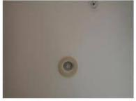
Corrections Recommended: The light fixture(s) at the entry area failed to function using the normal operating controls (unusual nose when switch is on). The bulb(s) in this fixture may be burned out. If the bulbs are not burned out, the condition of the fixture and wiring should be verified. We recommend repair as necessary to restore the function of this fixture.
