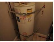
Corrections Recommended: The water heater strapping was installed in a manner that did not meet the states architects or water heater strapping kits manufactures installation instructions. We recommend repairing the condition noted. Corrections Recommended: The water heater was double strapped, it was not stabilized/blocked at the back to resist movement required by the states architects. We recommend repairing the condition noted.
