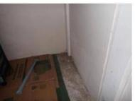
Corrections Recommended: Moisture stains were noted on the garage interior wall(s). The area appeared dry during the inspection. Repair as needed.
