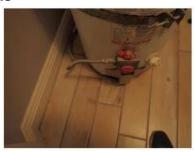
Corrections Recommended: A pan was not provided at the bottom of the water heater to prevent water damage in the event of a leak. Repair as needed.
