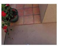
Safety Concern: Uneven surfaces (not flush) on the walkway at the front area. This condition is a trip hazard. Repair as needed for safety.
