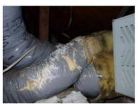
Corrections Recommended: There were air ducts with damaged/deteriorated outer plastic covering. This condition can effect the energy efficiency.
