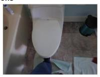
Corrections Recommended: The toilet is loose at the floor at the at the upper back left bedrooms bathroom. This condition can cause leakage and moisture damage. Repair as needed.
