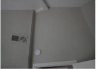
Safety Concern: Smoke alarm was installed too low at the upper back left bedroom. Smoke alarms should be installed in it's proper place and tested at regular intervals per the manufacturers instructions
