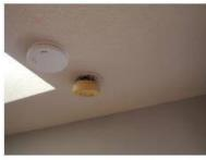
Corrections Recommended: The smoke alarm is hanging from it's wiring at upper hallway . Smoke alarms should be installed in it's proper place and tested at regular intervals per the manufacturers instructions
