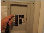
Corrections Recommended: A number of breakers/fuses in electric sub panel in the laundry room were not labeled to identify their use. All circuit disconnecting devices should be accurately labeled to allow the appropriate circuit to be shut off for maintenance or emergencies.
