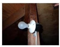
Corrections Recommended: The light fixture(s) in the attic failed to function using the normal operating controls. The bulb(s) in this fixture may be burned out. If the bulbs are not burned out, the condition of the fixture and wiring should be verified. We recommend repair as necessary to restore the function of this fixture.
