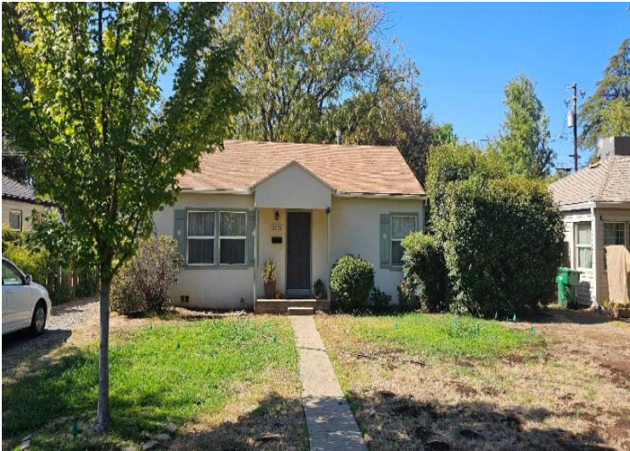
Front of the structure.
