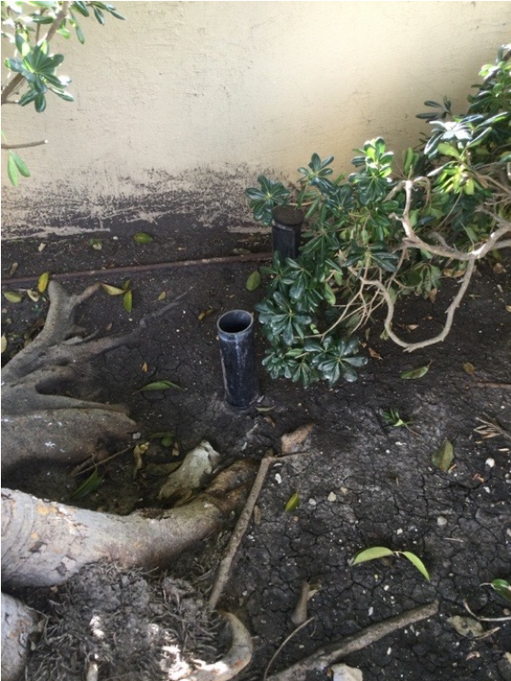
Planter behind the front wall.
