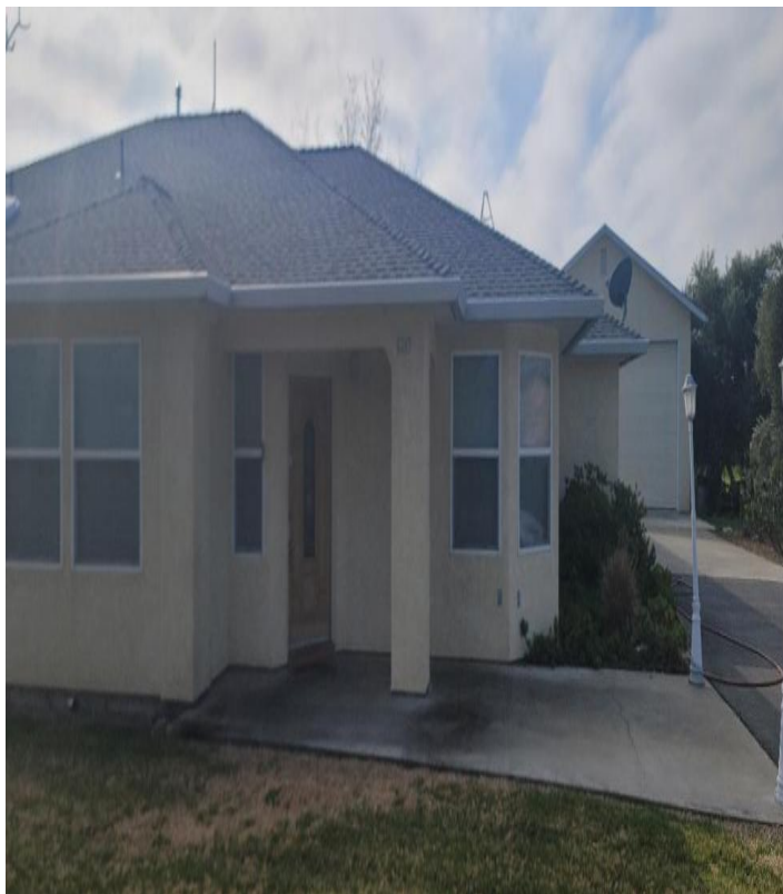
Front of the structure.
