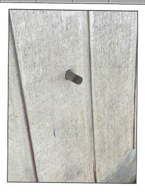
25. Condition: • Improper TPR drain material used. Material is to be the same as allowed for water distribution. (galvanized steel, hard-drawn copper)no flexible line.
