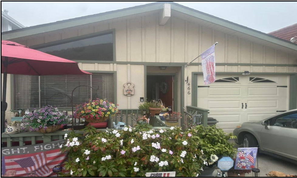
FRONT VIEW OF SUBJECT PROPERTY
