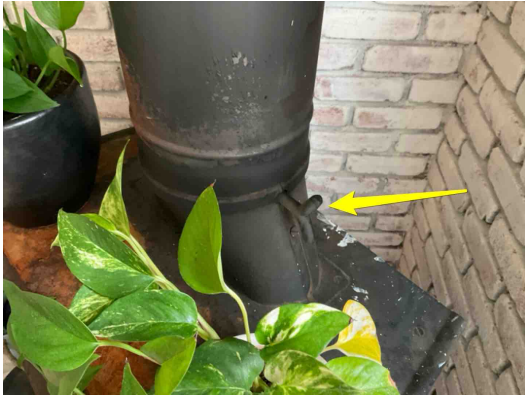
Functional damper on a fuel burning appliance
