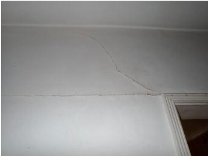
This shows a crack that was a concern to the client. This is the door frame between the kitchen and dining room.
