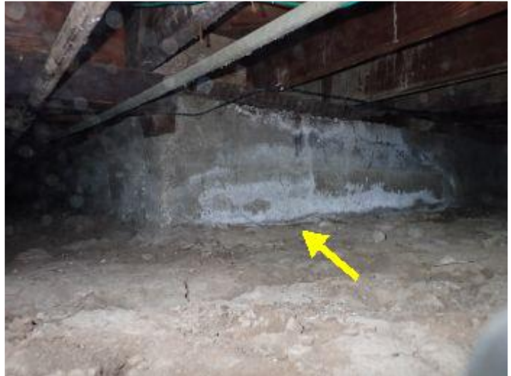
FYI: There are areas of efflorescence observed. This is a mineral deposit left behind from exterior water infiltration or standing water from plumbing leaks, etc.
