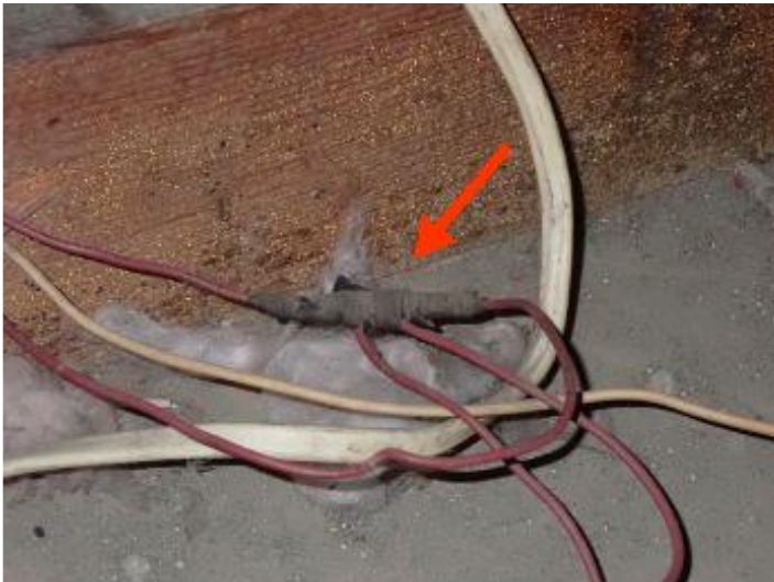
*Exposed wire splices were visible in the attic.
