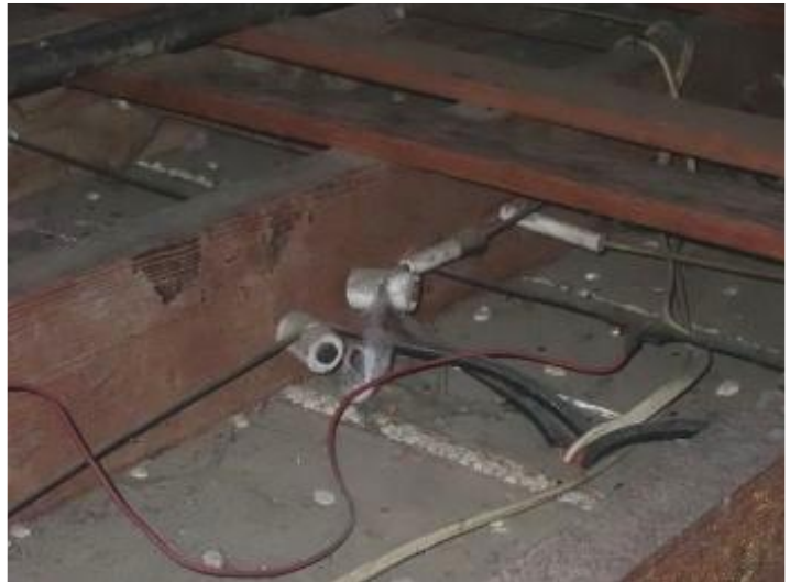
Live knob and tube wiring present.
