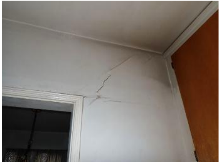
This is the same door frame from the kitchen side, showing the identical direction of small cracks.
