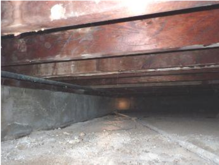
The general condition of the concrete perimeter foundation appears serviceable.
