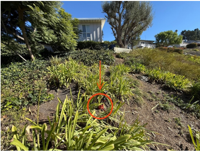
Furthest camera was pushed due to block in sewer line.
