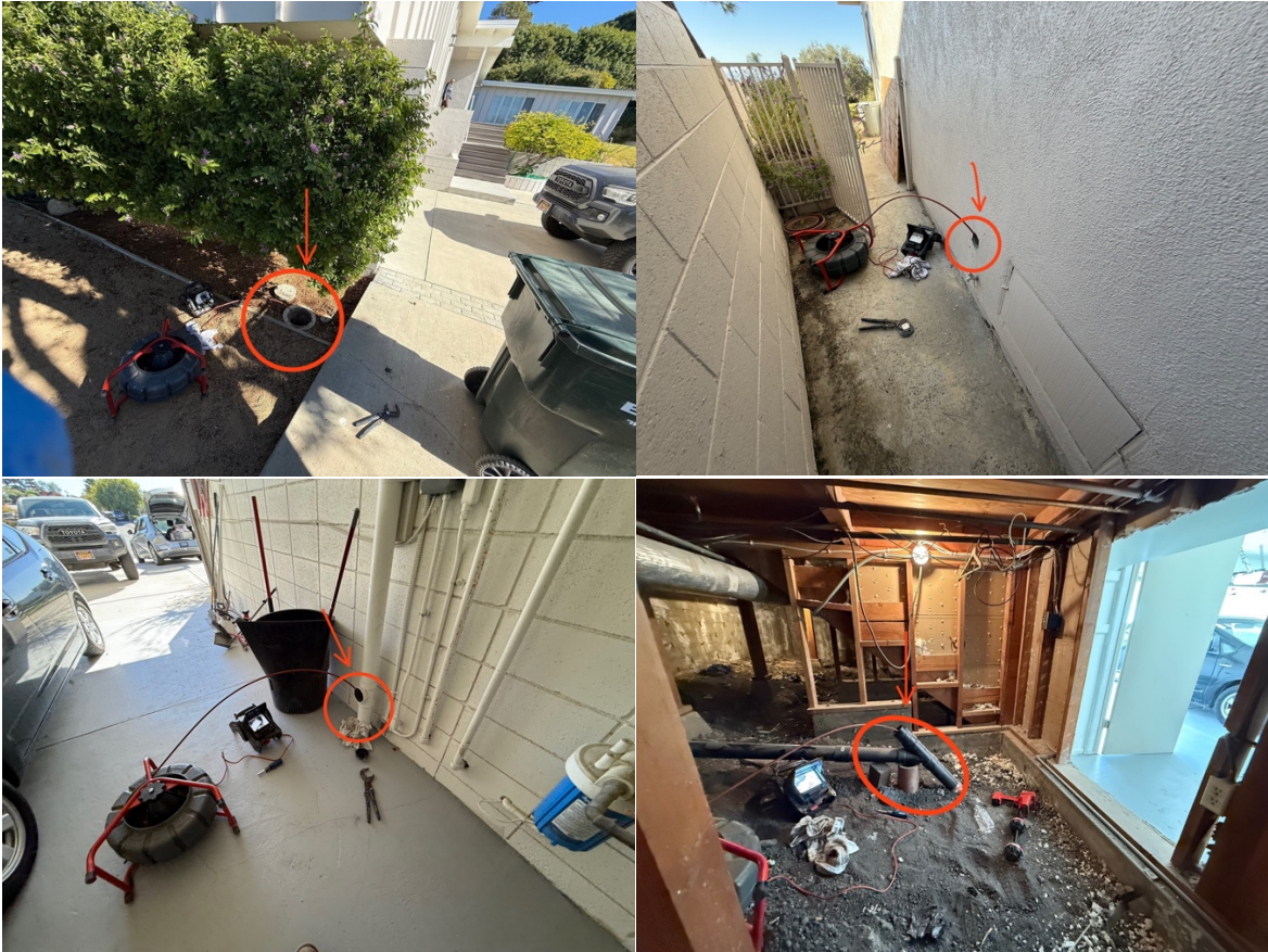
Location of cleanouts used for inspection.
